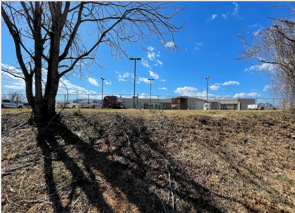
The rear of the existing detention center.
