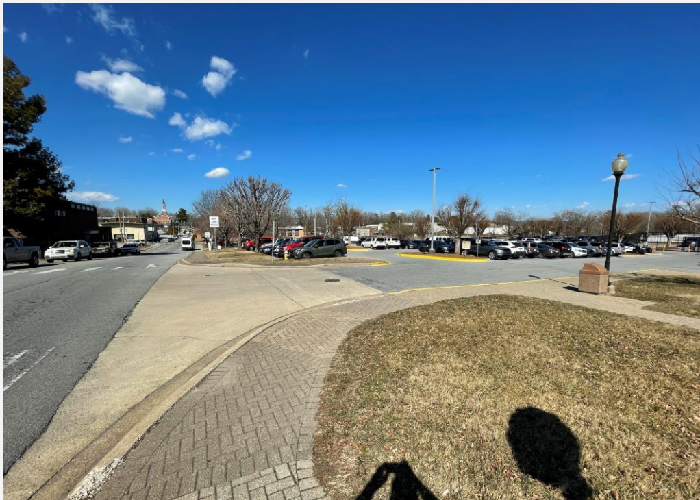
The existing courthouse parking lot entrance, located across from 3rd Ave and to be retained, will be used as part of the public drop-off area in front of the new courthouse.
