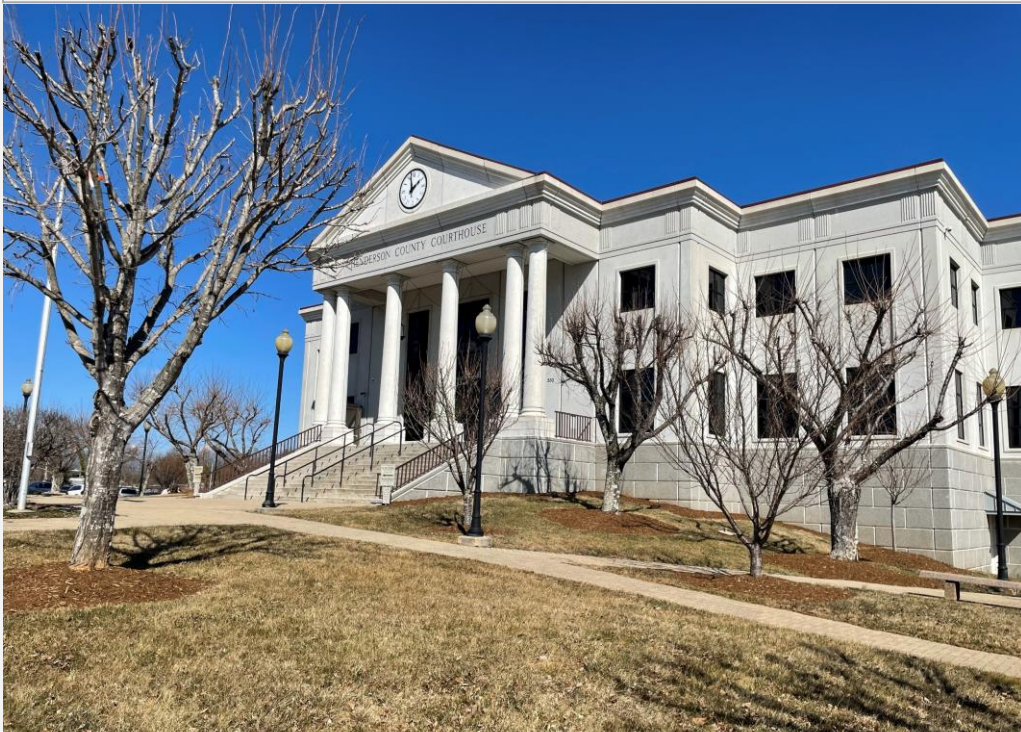
View of the 1995 courthouse.
