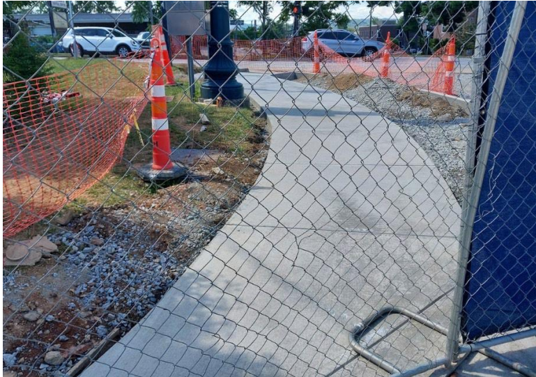
CO 19. Completed sidewalk at intersection.
