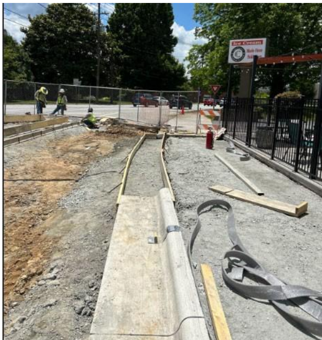
CO 9. Forming for concrete to be placed at Creamery.
