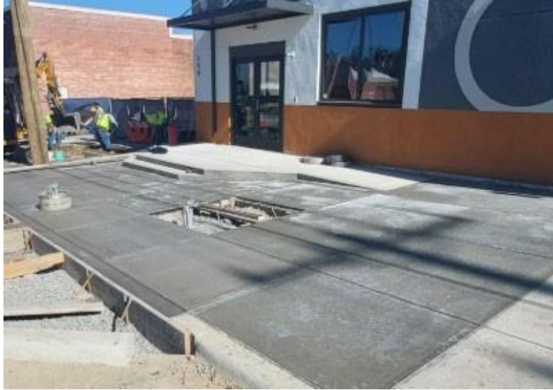
CO 1008. Ramp, landing, and steps at Mission.
