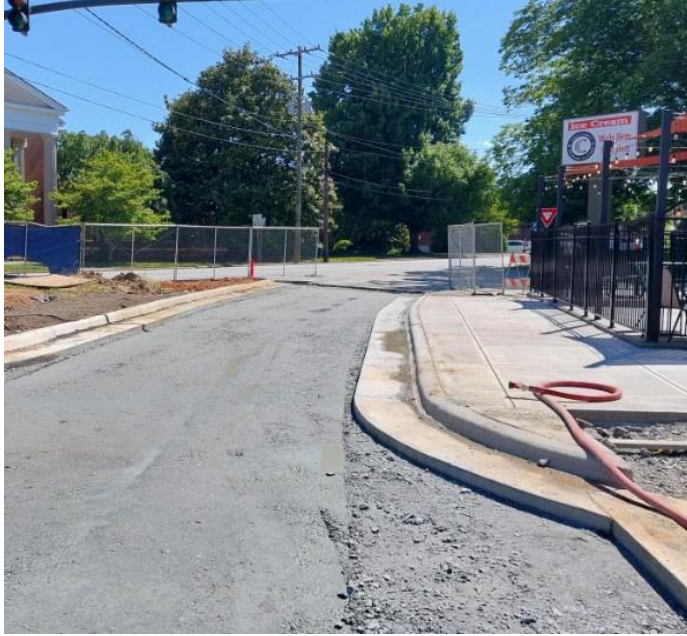
CO 9. Finished sidewalk at the Creamery.
