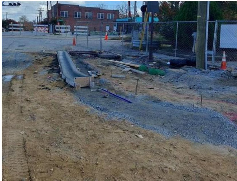
CO 1008. Tie in work at railroad tracks.
