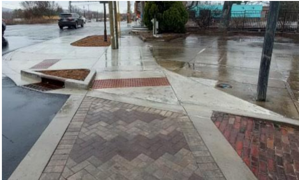
CO 1008. Completed work at railroad tracks.
