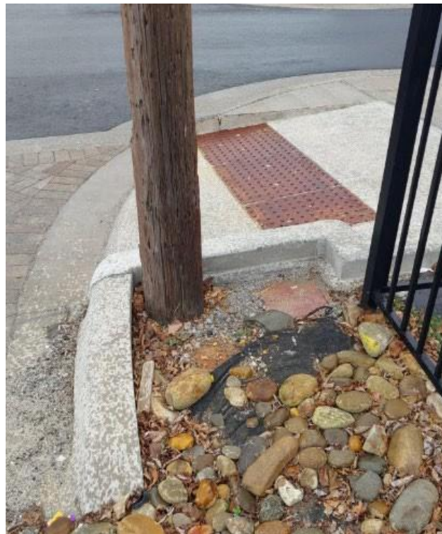
CO 16. Relocated utility box at the corner of N. Grove.
