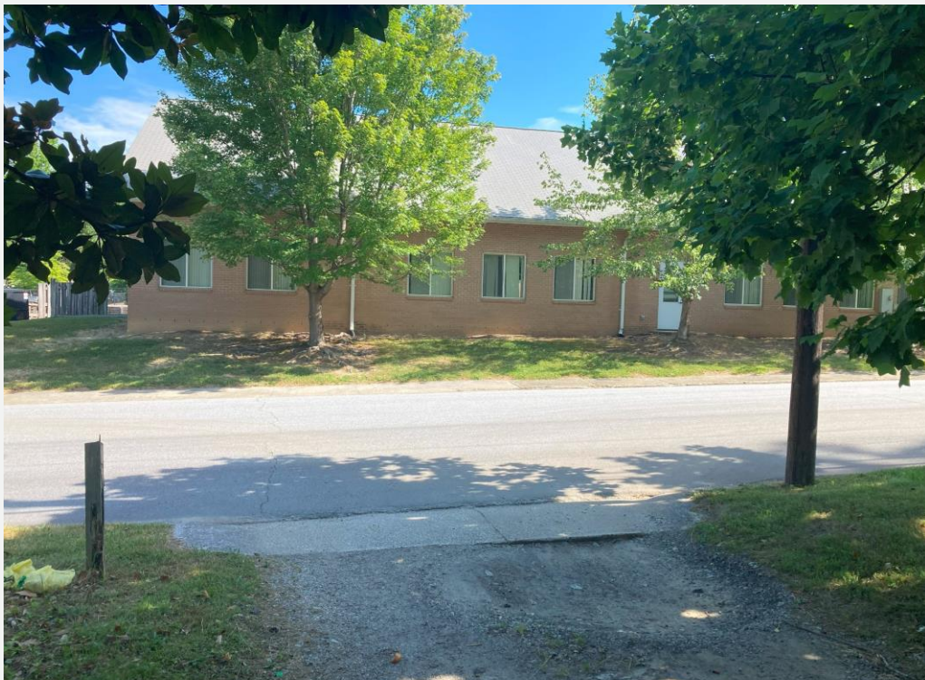
View of 1st Church of the Nazarene and 1st Ave from frontage of subject property
