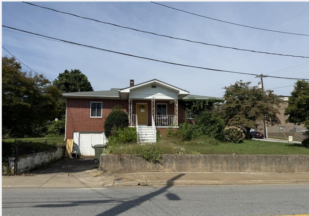
View existing house from S Grove St.
