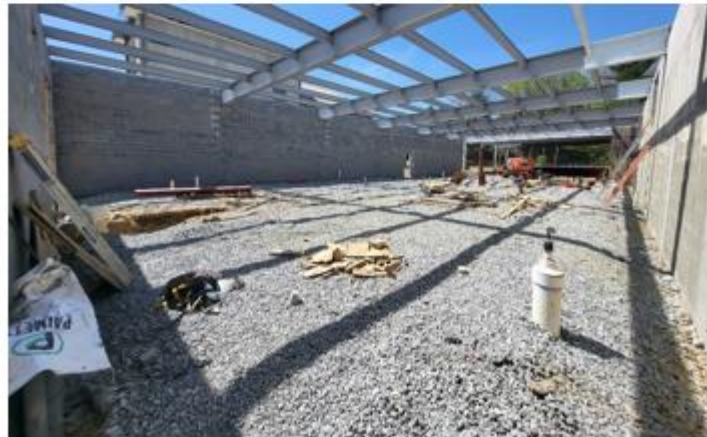
Biosolids Thermal Dryer Facility Construction. April 2026.
