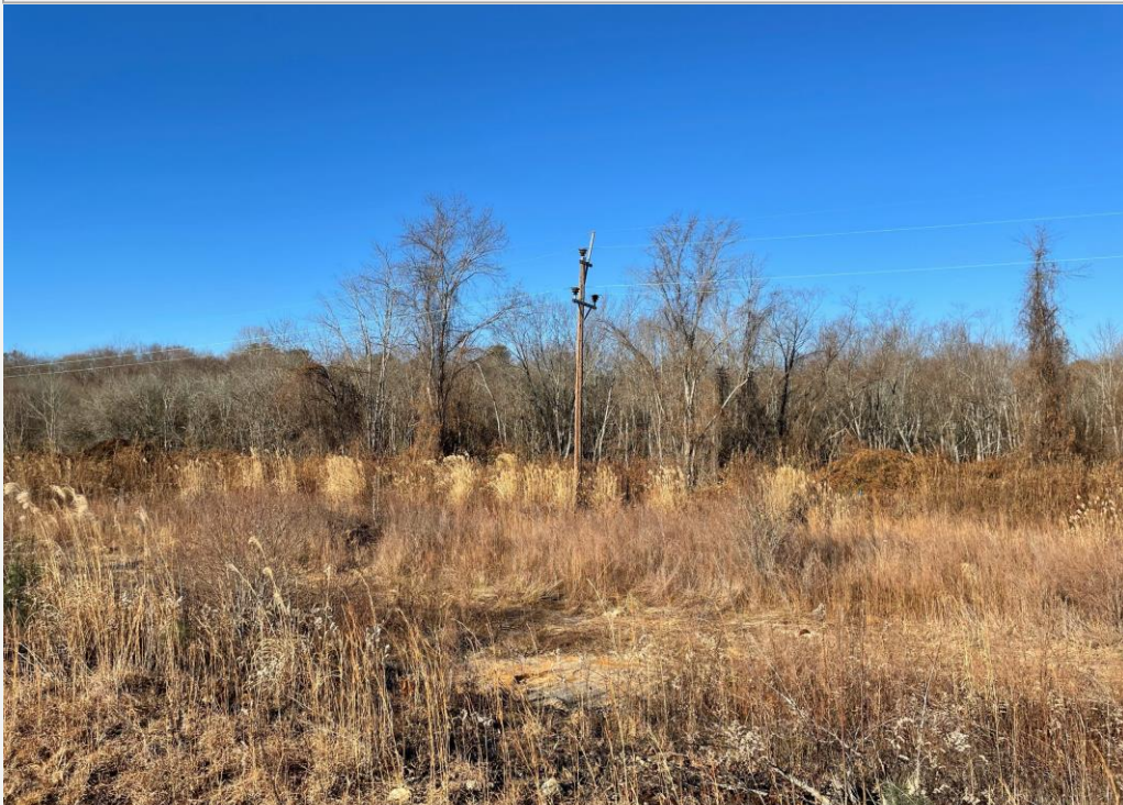
View of existing power lines that are associated with the utility easement on the north side of the site.
