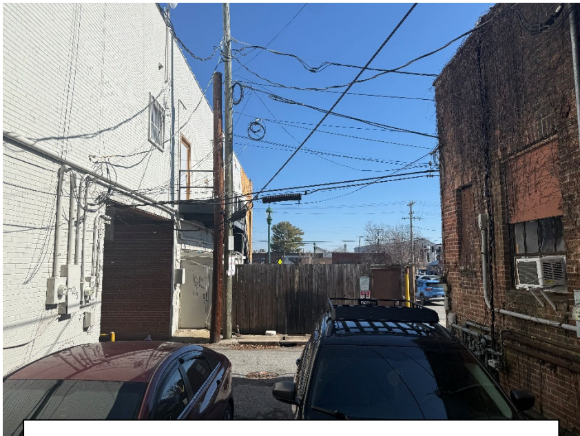
View of current rear parking area from back of building, showing proposed stairwell impacts.
