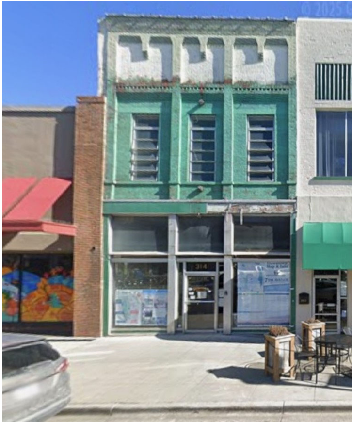
Existing front façade of 314 N Main Street.
