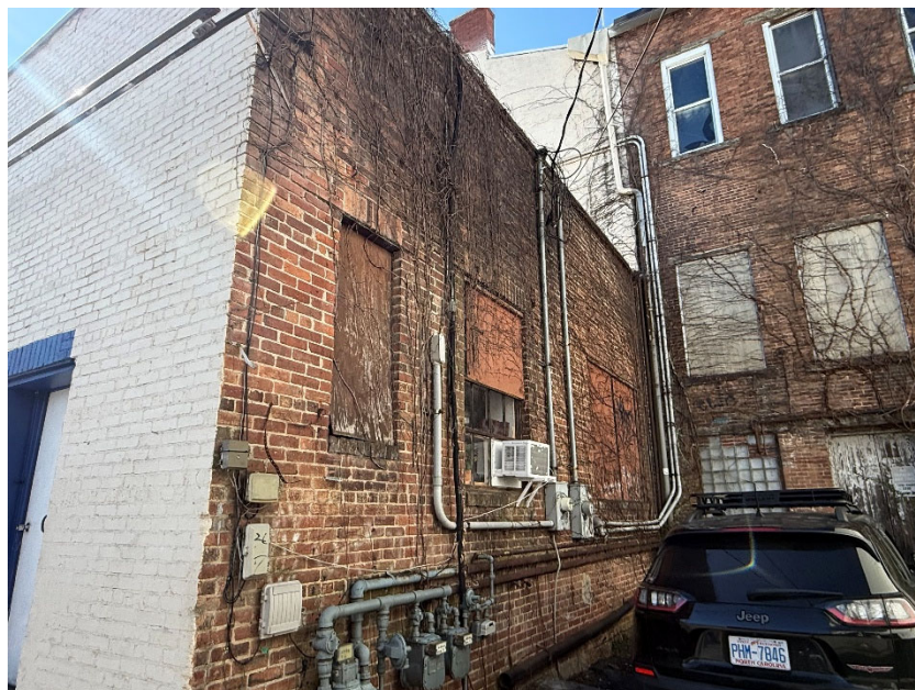
Neighboring building stairwell addition will border
