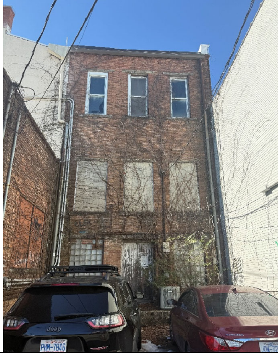
Current rear façade
