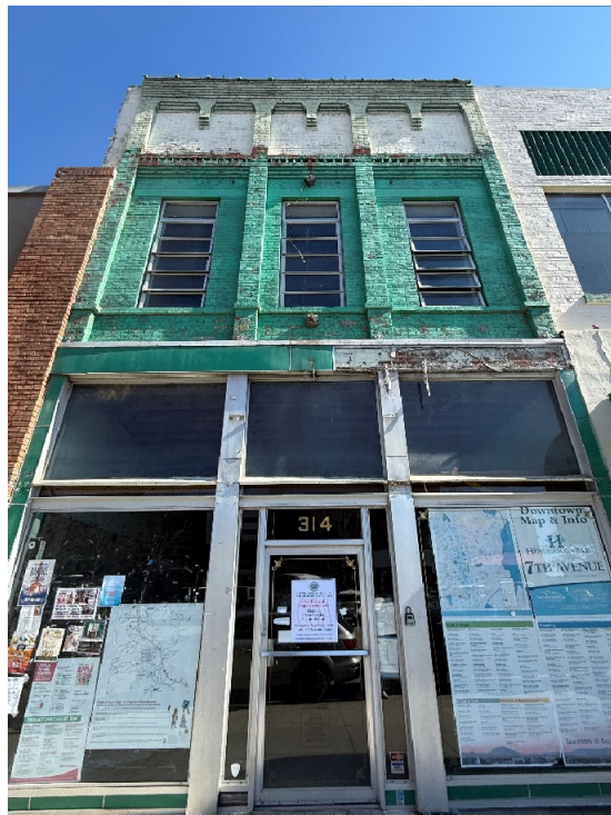
Close up photo of storefront facade
