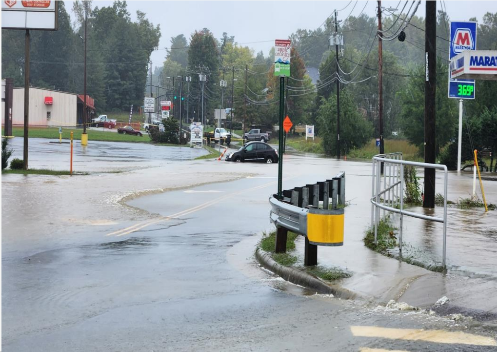
View of Greenville Highway during the rain event before Helene (9-26-24)
