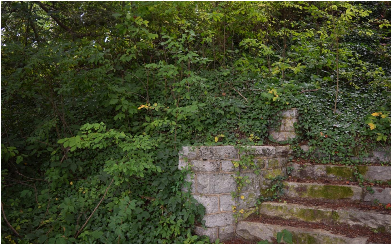
13. Staircase at rear of spring, view southeast
