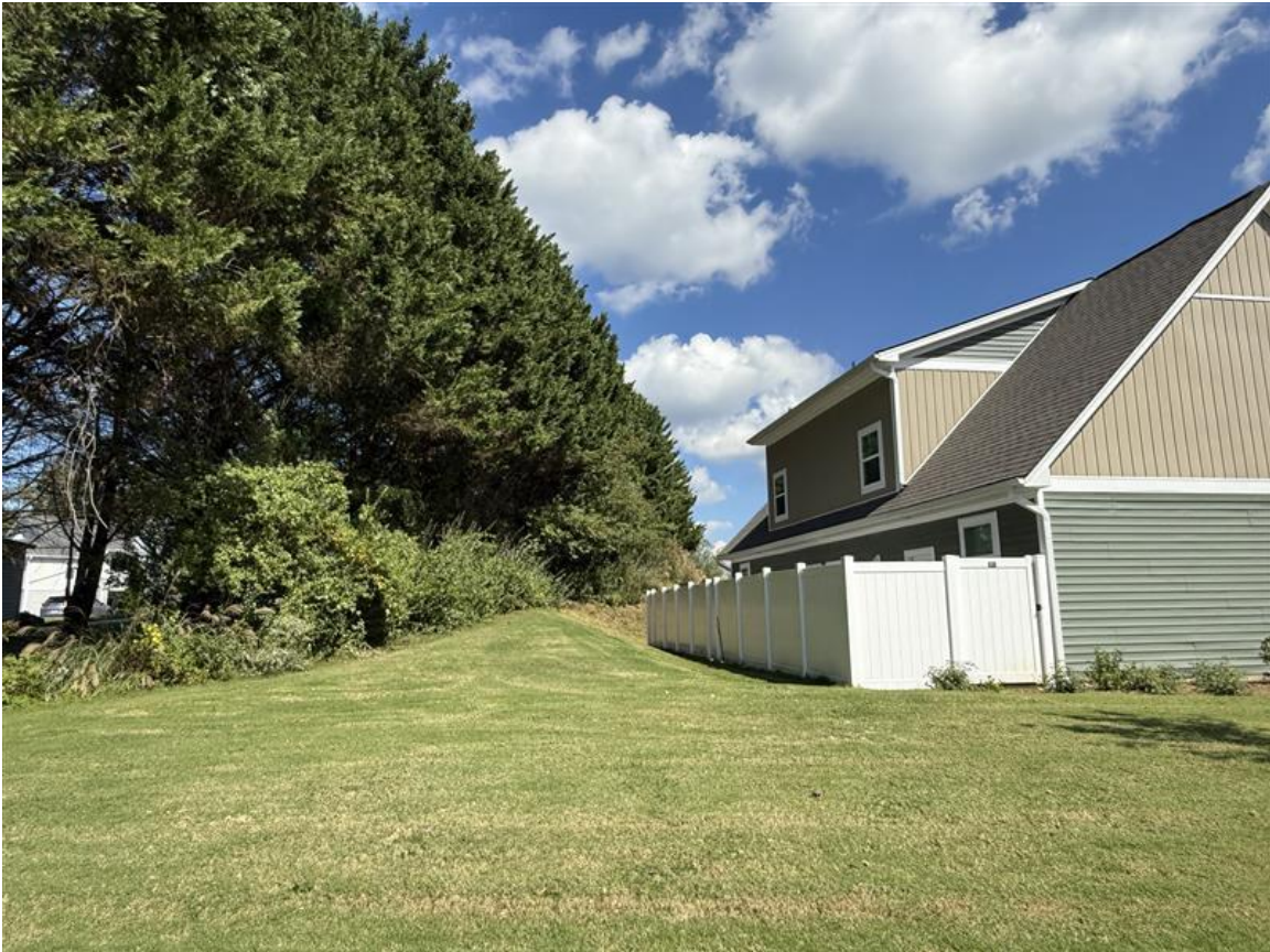
Photo 1: View north east at corner of building encroaching into setback. Note that the City of Hendersonville does not regulate fences, so there is no encroachment request needed for the fence.
