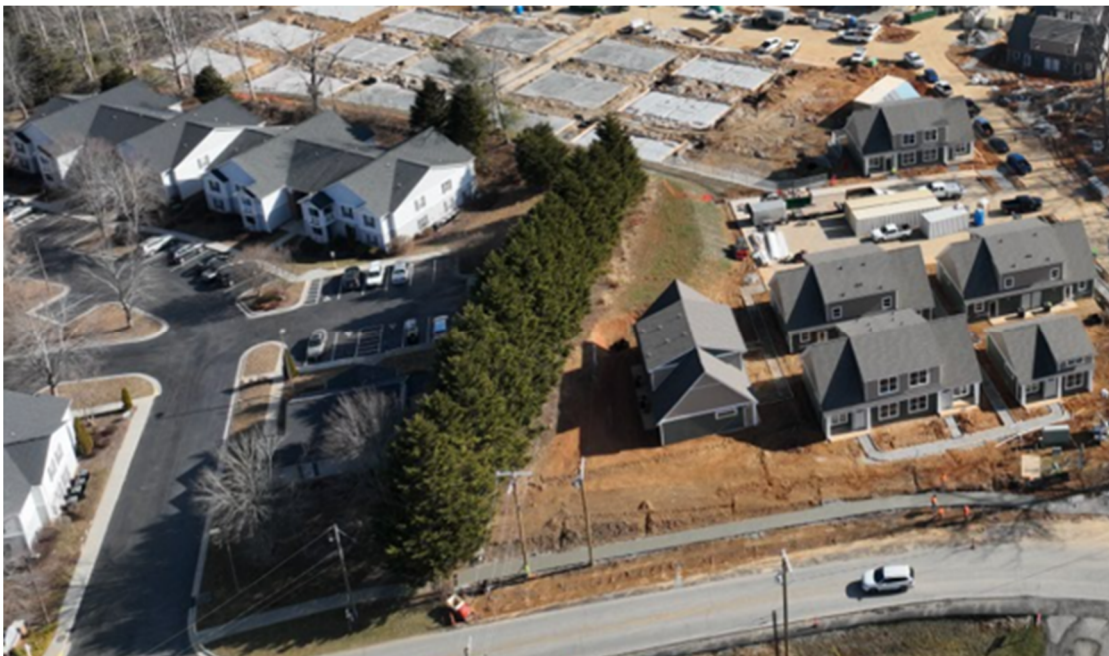
Picture of unit and buffer plantings on adjacent property during construction.
