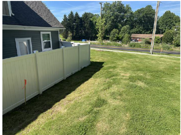
Setback line stakes on the opposite side of the building
