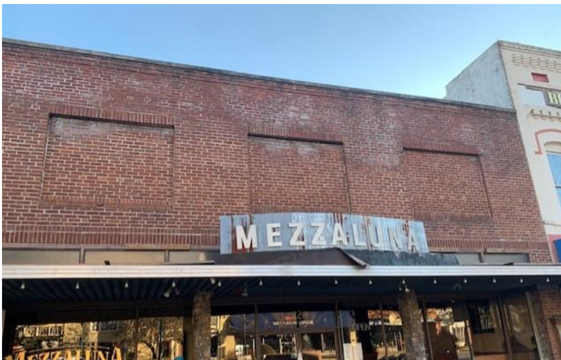
226 N Main St.: Non-contributing one-story brick building. The 2005 Local Designation Report does not describe the upper façade windows as at the time the survey was conducted the upper façade was covered with a modern corrugated metal façade that was later removed in 2008. There is no indication on the condition of the windows after the façade was removed.
