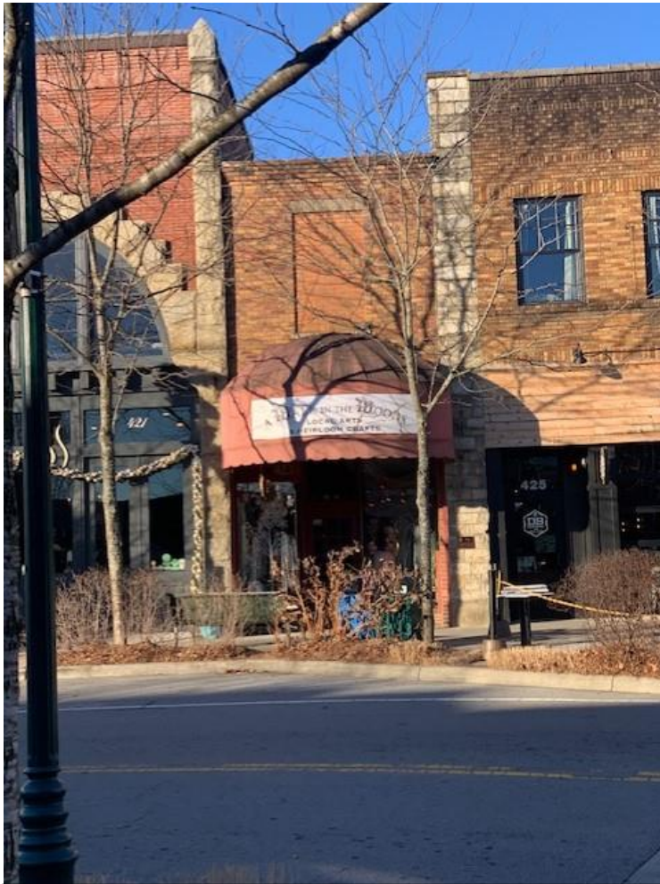
423 N Main St.: Contributing, one-story brick commercial building and bricked-in second story. Example of in-fill brick on the second story that does not match the existing brick façade.
