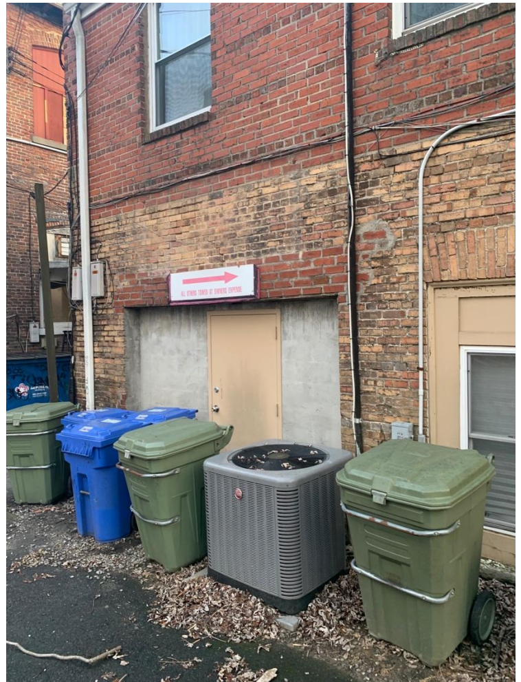
Example of mismatched brick on rear façade of the building the subject property is located in.
