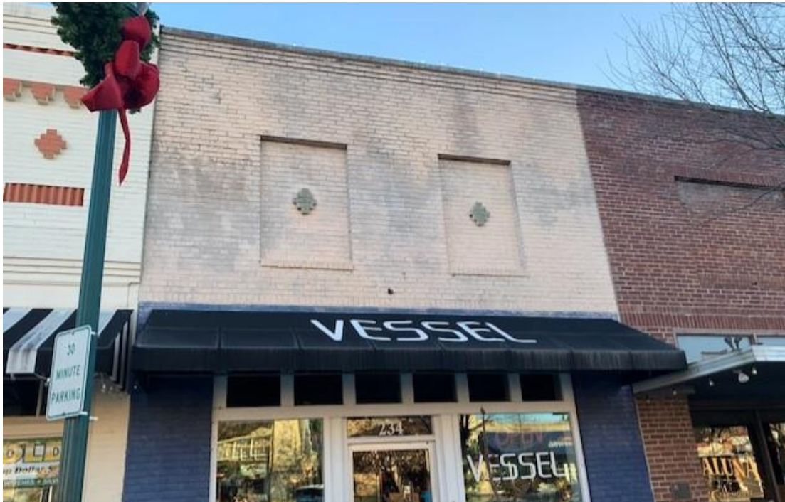
234 N Main St.: Early 20 th century two-story painted striated brick commercial structure. The second-story windows have been filled in with brick panels with diamond ornament.
