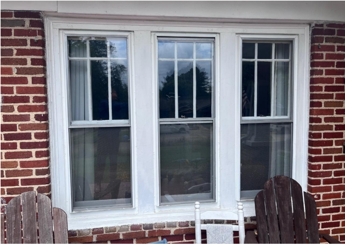
Appendix A 9: Set of 3 wood cased 6 over 1 windows featuring 3 small lights over 3 vertical lights over 1 single pane
