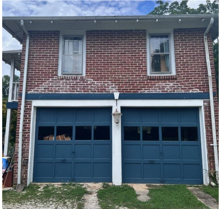
Appendix A 15: Original sectional overhead garage doors featuring 4x4 panels with 4 panes across upper-mid section
