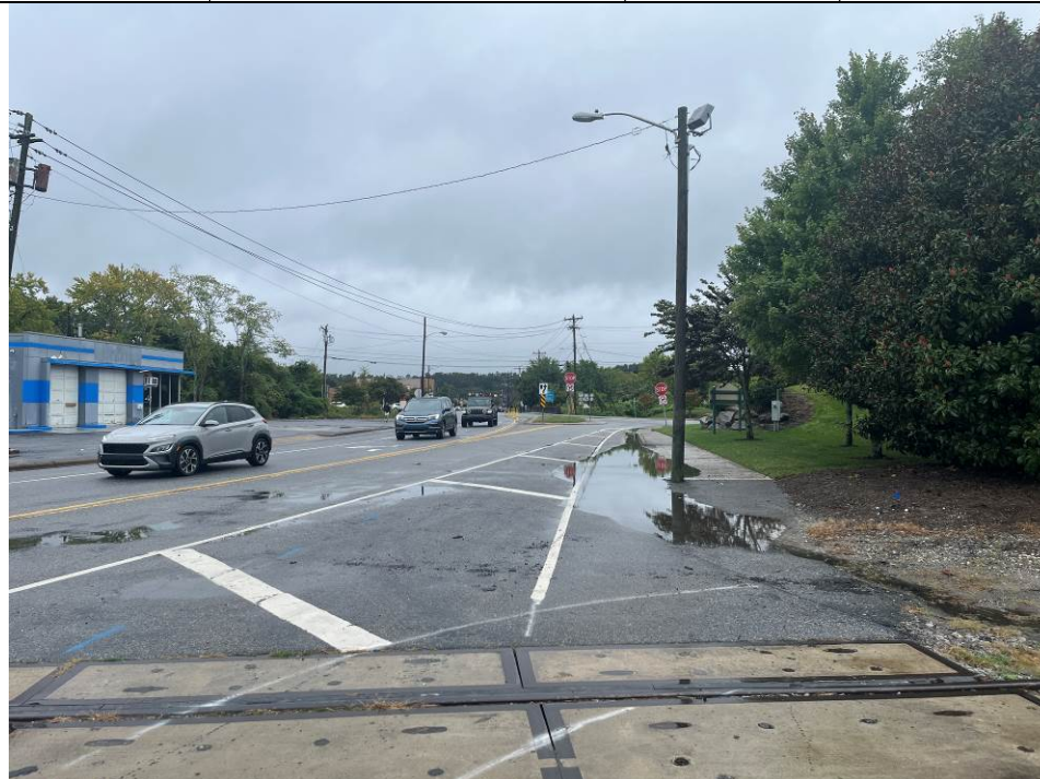
Looking S along subject's frontage along S Main St.
