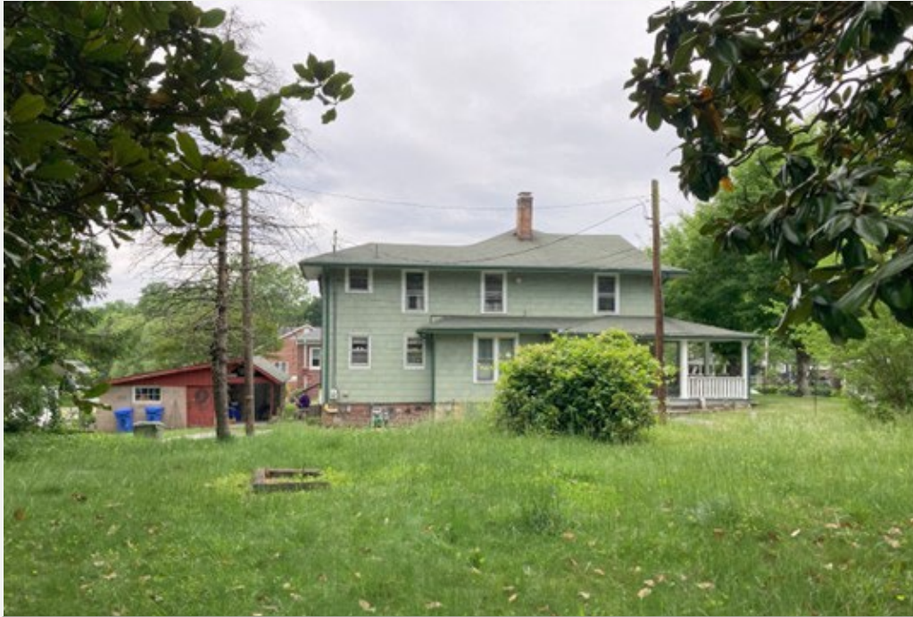
View of adjacent property to the west.
