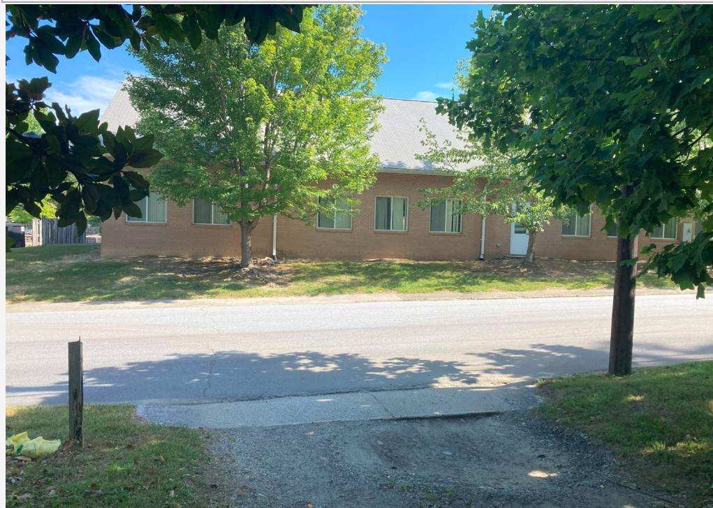
View of 1st Church of the Nazarene and 1st Ave from frontage of subject property
