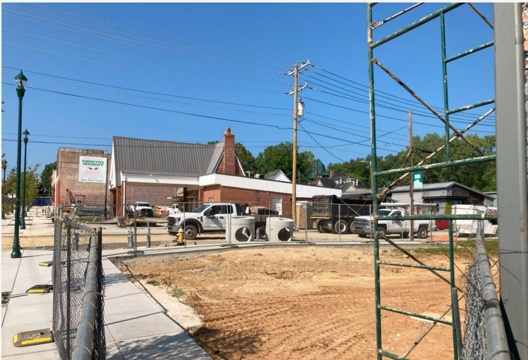
View of corner of 7 th Ave and Locust St - empty lot where existing building was recently demolished.
