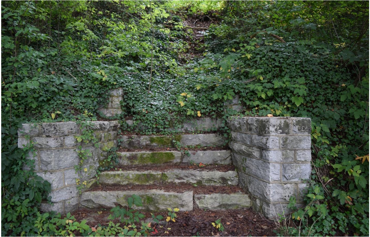
12. View of stairs, cheek walls, and hillside, view southwest
