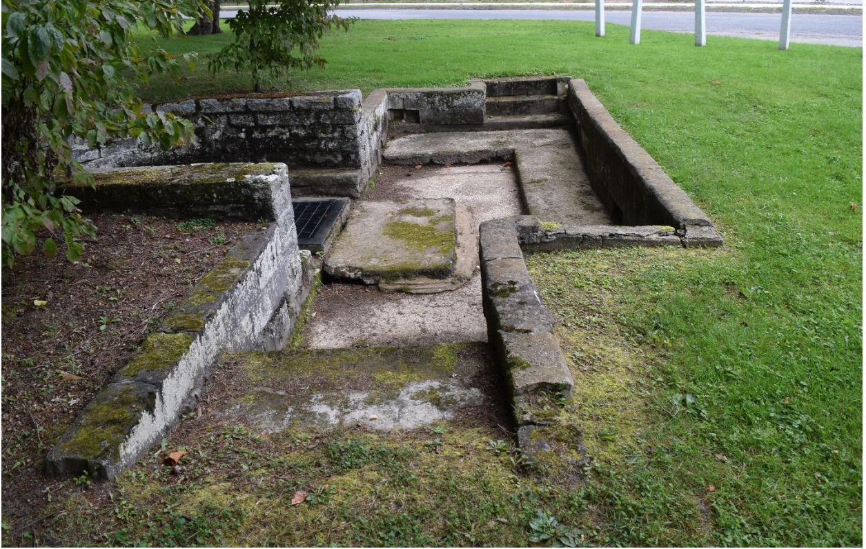
9. Lenox Spring stonework, view northwest
