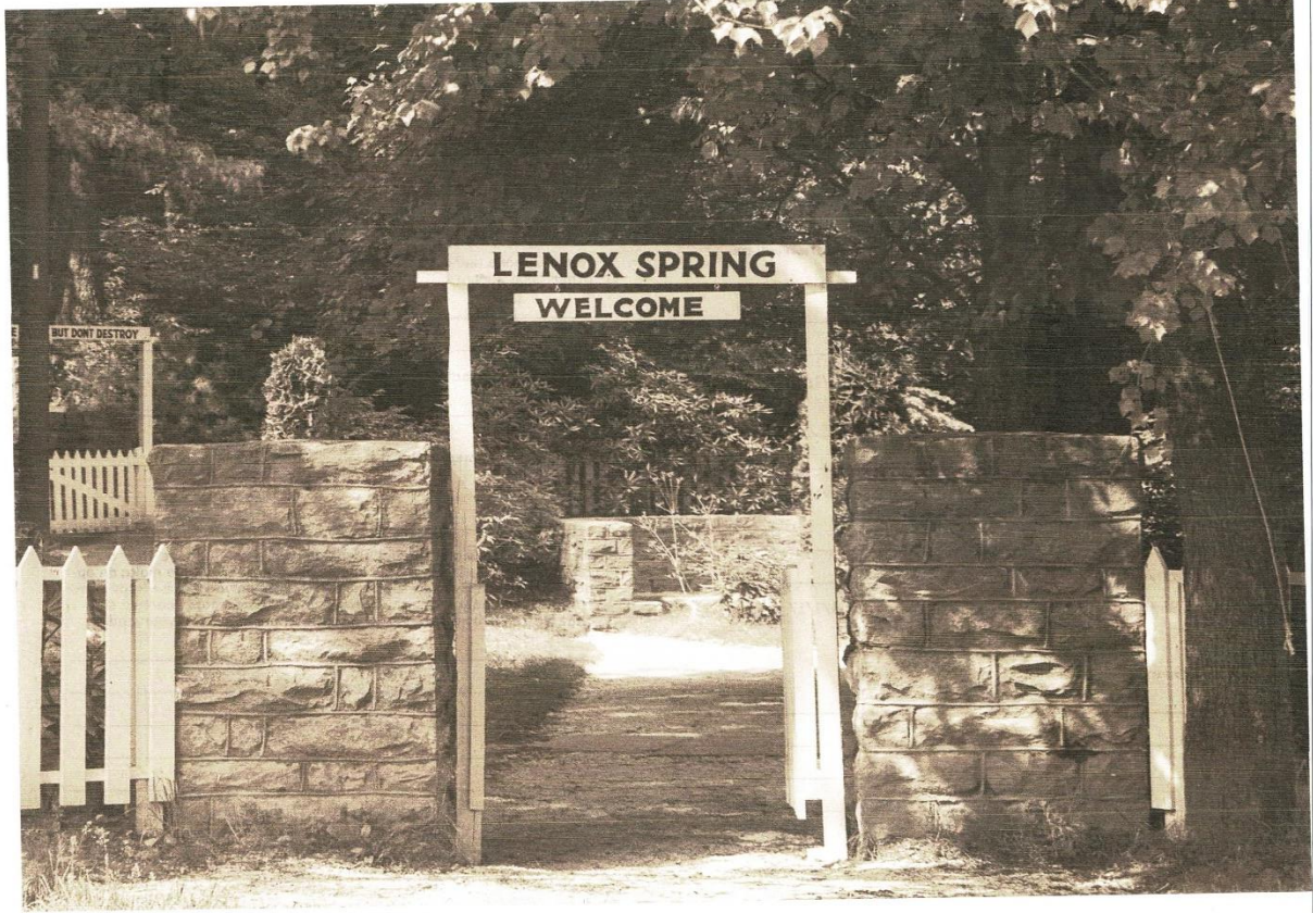
Lenox Spring Documentary Photo, date unknown, details of entry, piers, fence, and wall at spring
