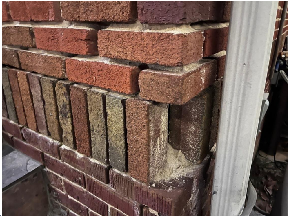
Appendix A 39: Portions of the brick facade need repointing. Also visible in photo is the distinction between the brick used for foundation and brick used for façade
