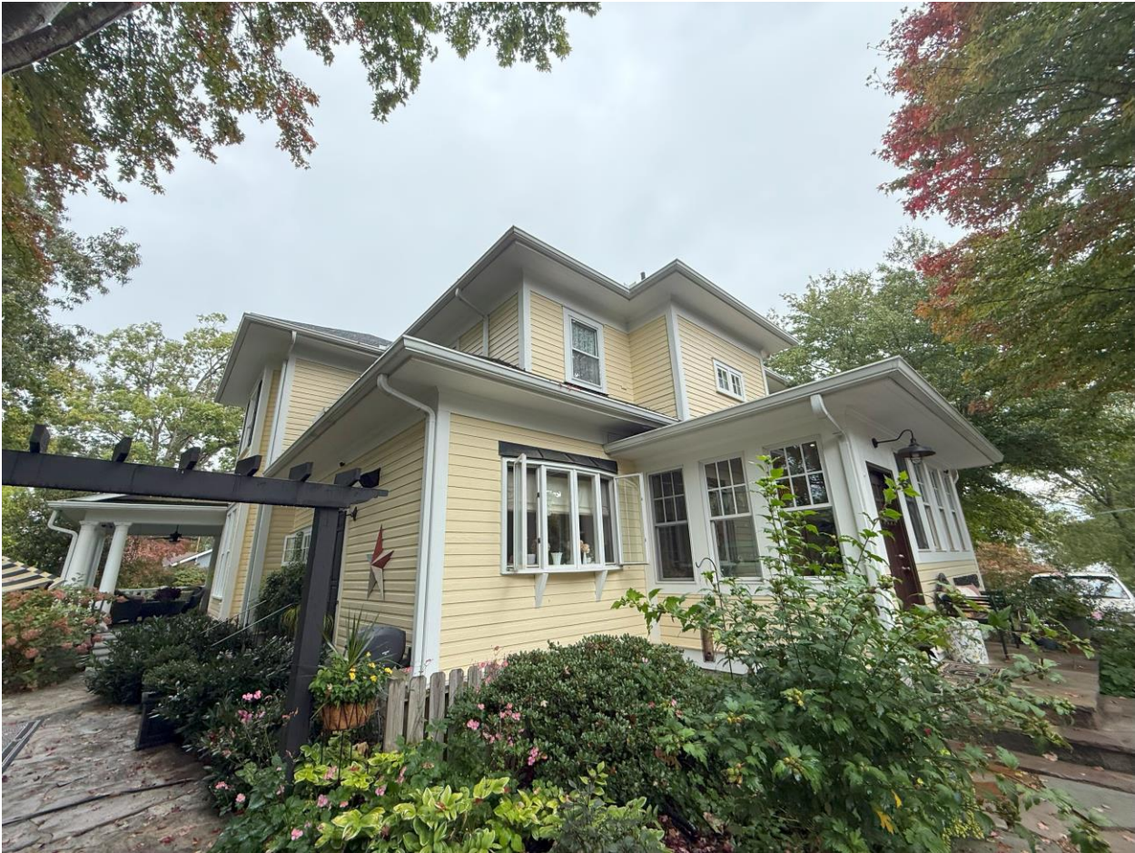
Fig. 7: Rear of property. Rear addition was added to the property
