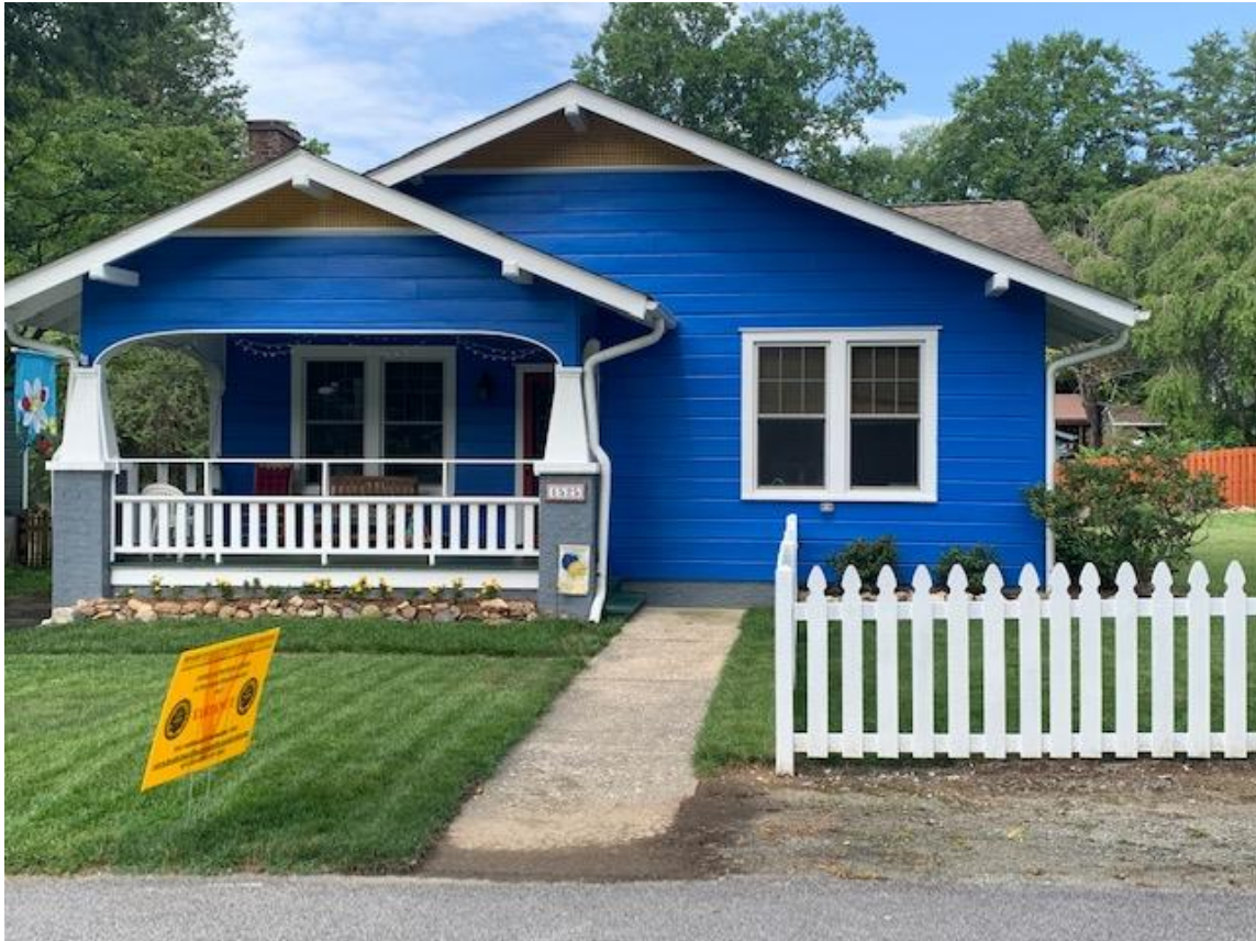
Exhibit C – Site Photos B22-070-VAR 1525 Ridgewood Blvd
