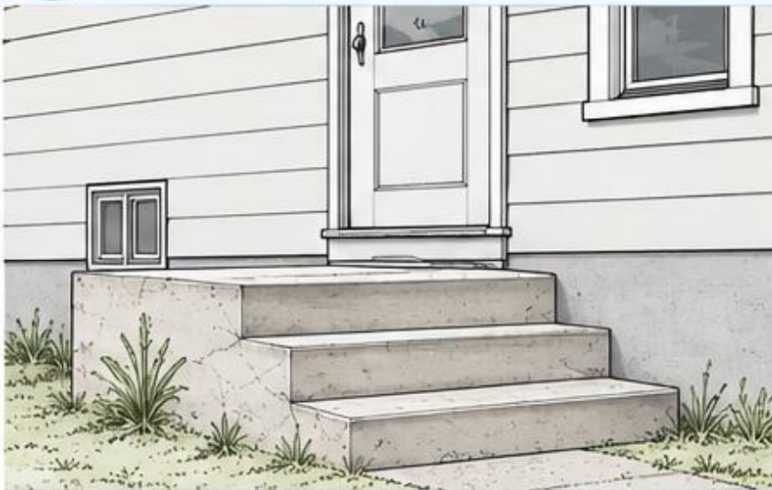
Existing concrete side landing and steps.
