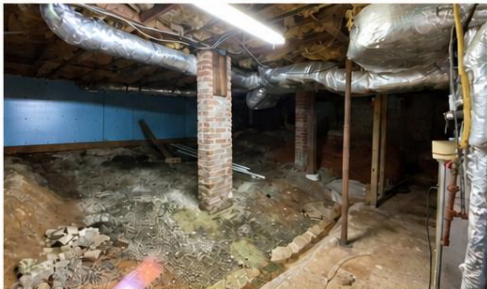
Existing crawl space showing masonry piers and soil floor.
