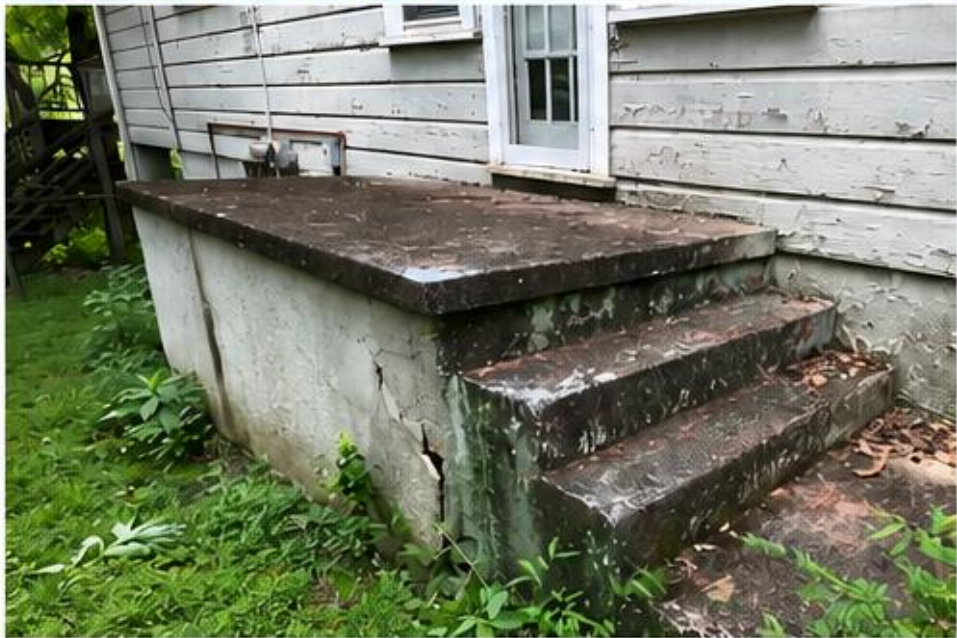
Existing concrete steps and platform to be removed.
