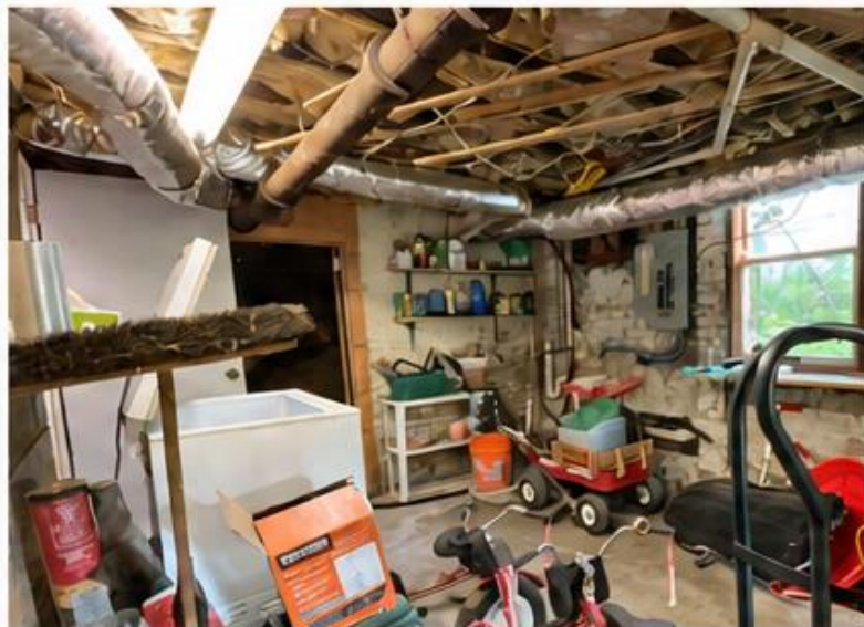
Existing basement showing masonry walls and interior conditions.
