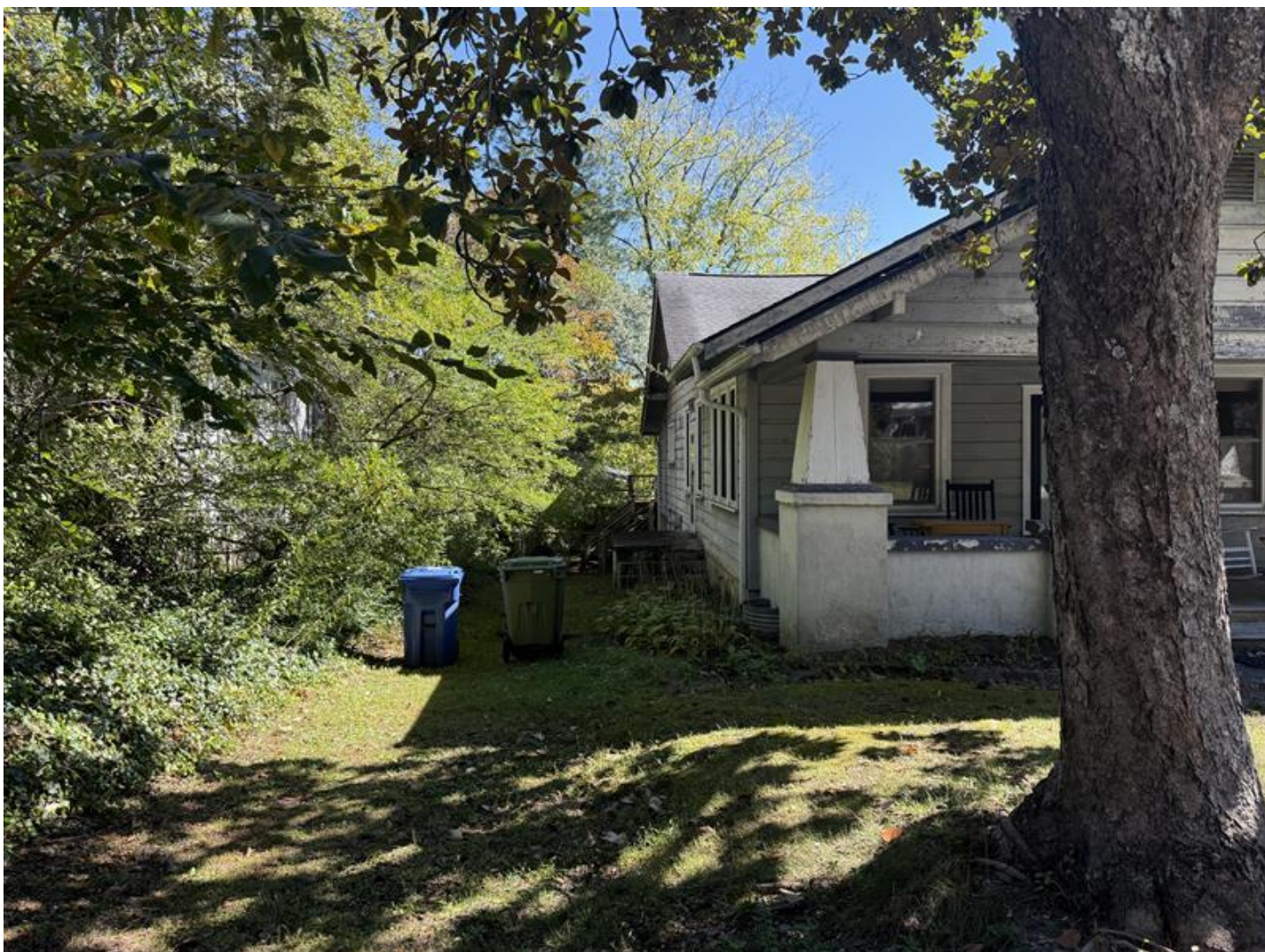
Photo 2 : View of subject property looking down the northern side of the property. The concrete porch and steps is proposed to be demolished and a wooden deck and steps is proposed.
