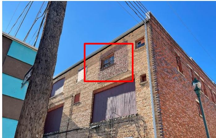
East side of building (rear). Red box indicates which window is proposed to be replaced.
