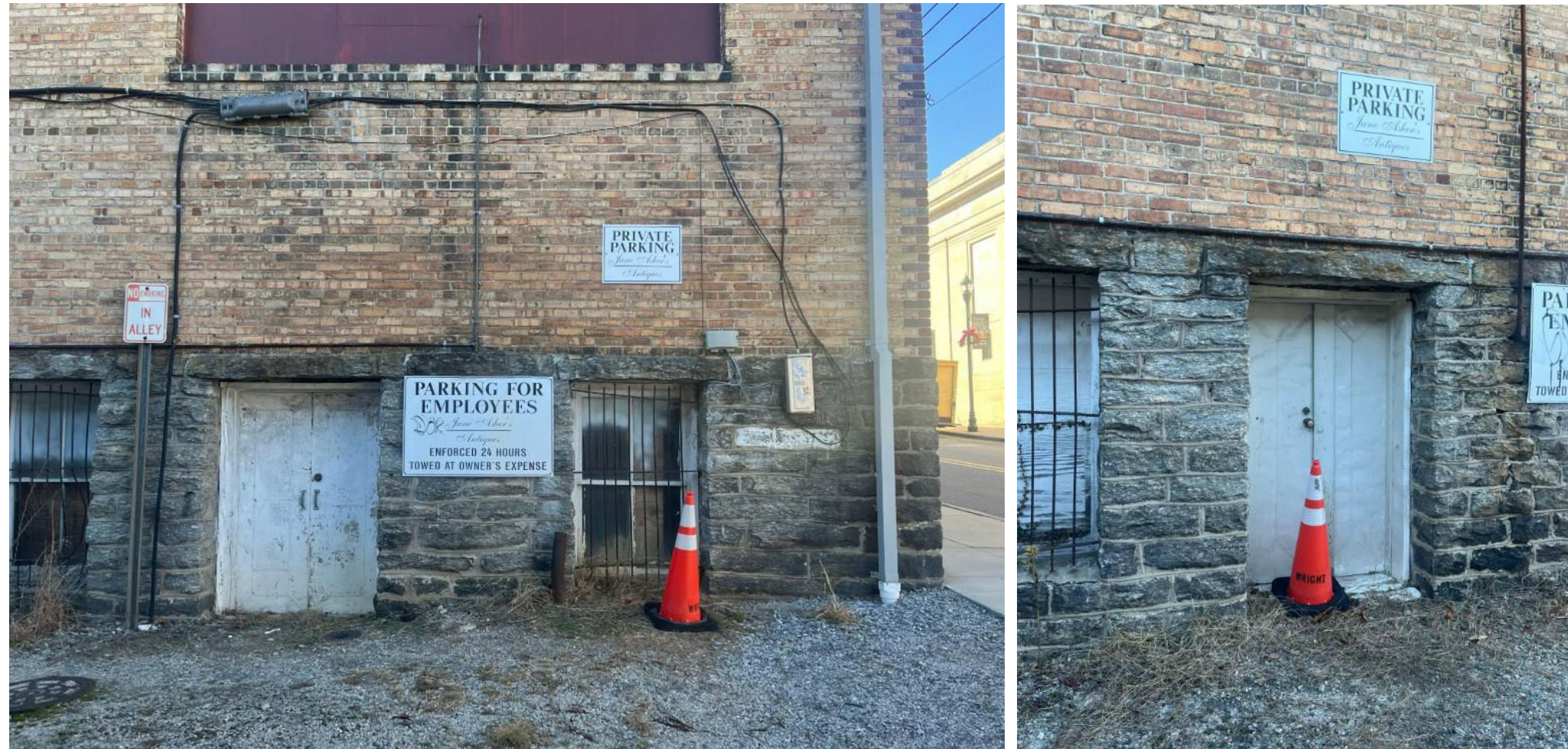
EXISTING PHOTO OF 344 MAIN ST BACK ALLEY VIEW
