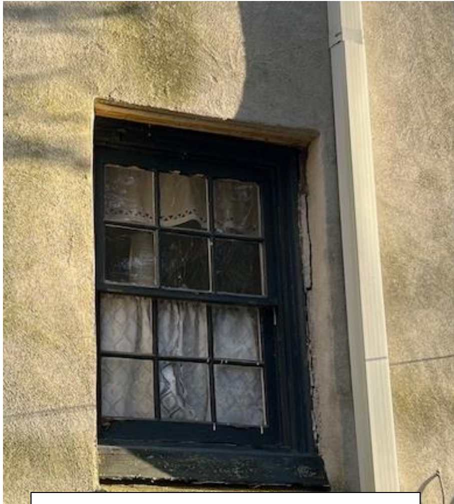
Exterior view of existing kitchen windows.
