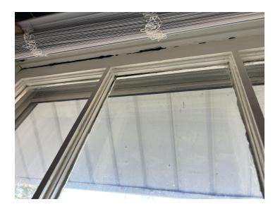
• There is extensive wood rot in many windows making their reconditioning near impossible. These rotten windows are not salvageable as they have extensive water damage and rot.
