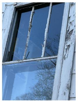
• Some windows have broken or cracked glass panels are are in need of immediate replacement.
