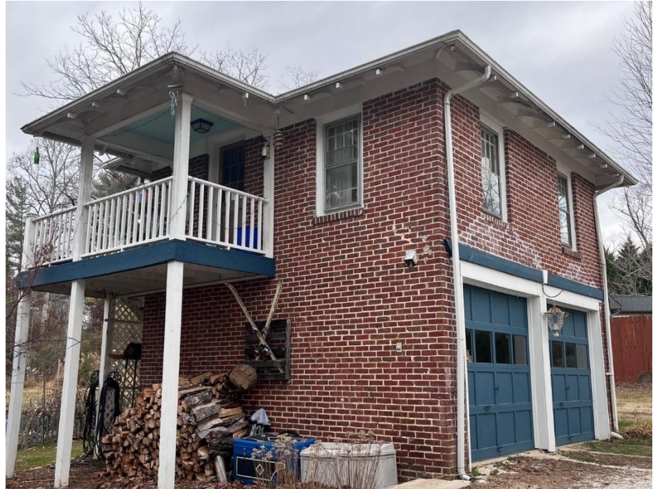
Appendix A 15: Original sectional overhead garage doors featuring 4x4 panels with 4 panes across upper-mid section
