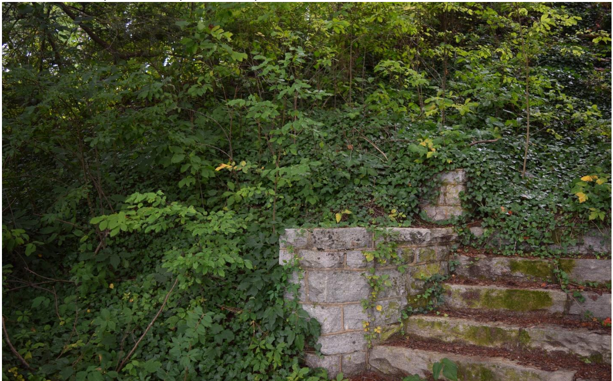
13. Staircase at rear of spring, view southeast
