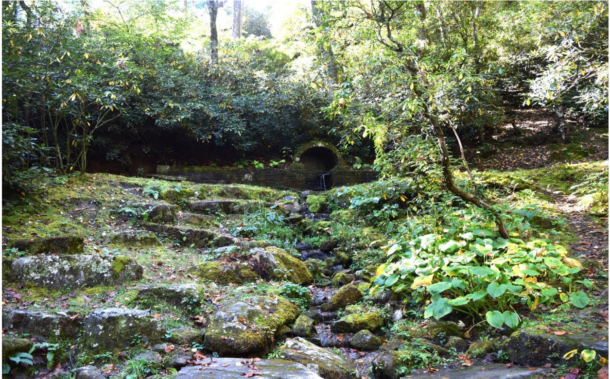
Crystal Spring and stonework, view southwest
