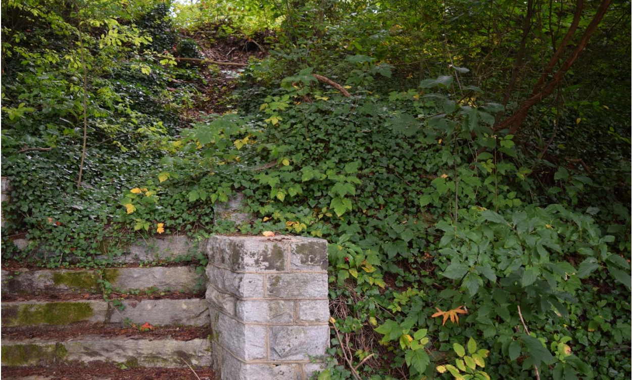
14. Staircase as rear of spring, view northwest
