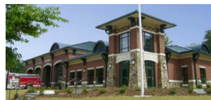
Waynesville Fire Station No. 1 Waynesville, North Carolina
