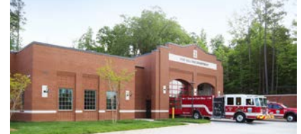
Fort Mill Fire Station No. 2 Fort Mill, South Carolina
