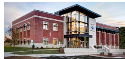
Garner Town Hall Garner, North Carolina
