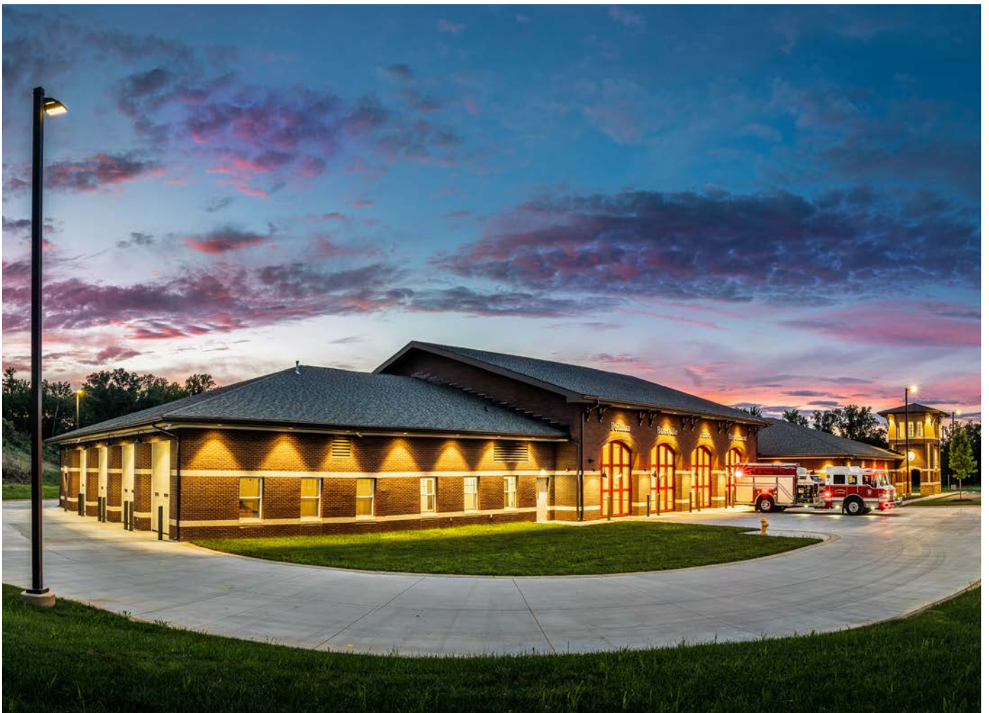
Pelham-Batesville, SC Fire Station No. 1 & Headquarters
