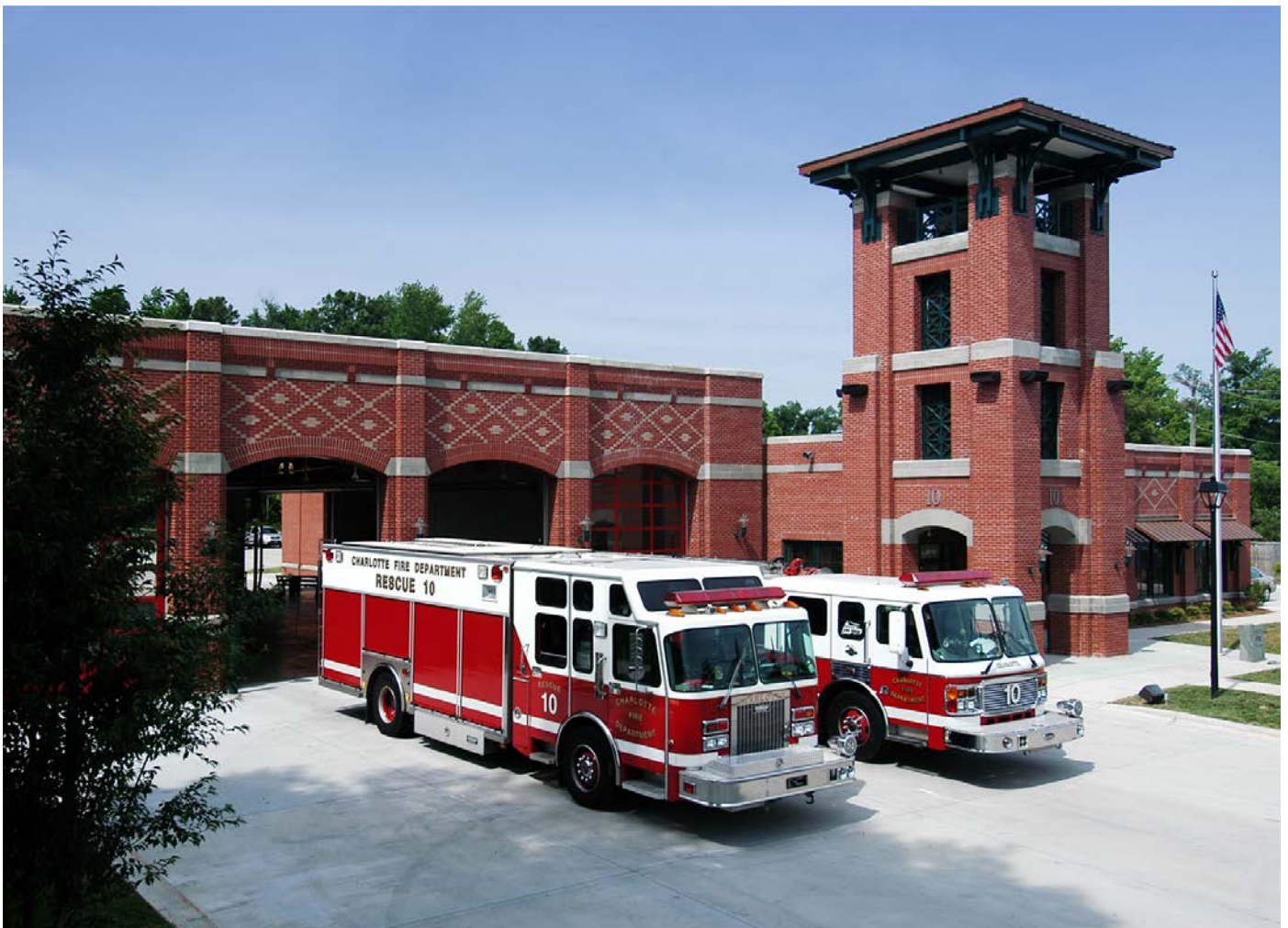
Charlotte Fire Station No. 10 (National Fire Station of the Year 2006 - Fire Chief Magazine)
