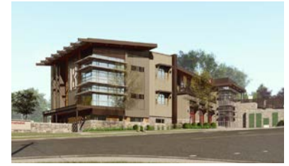
Asheville Fire Station No. 13
