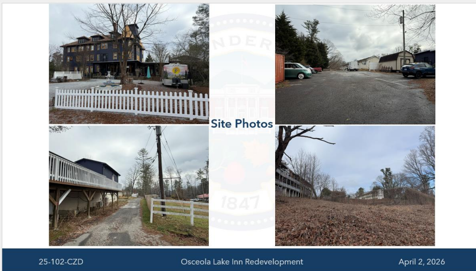
N Lakeside drive Applicant applied for and received a demolition permit to begin the demolition of the building seen in the left side of the bottom right image. The building is unsafe and therefore staff provided a demolition permit to assist with taking the structure down.
