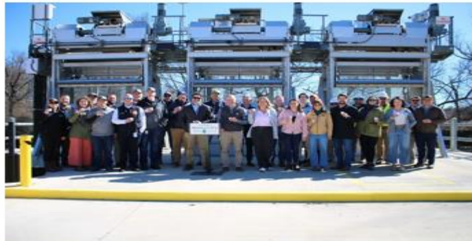
Elected officials, external partners, and utility staff celebrate the launch of the new French Broad River Intake. February 13, 2026.
