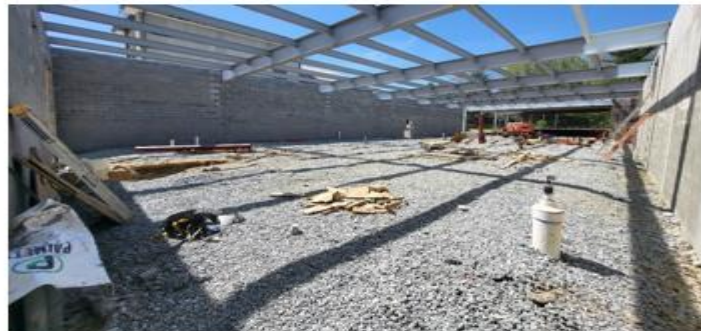
Biosolids Thermal Dryer Facility Construction. April 2026.
