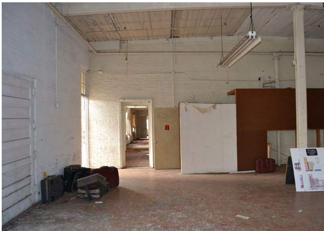
64. Grey Mill, 1919 Building, Looking West
