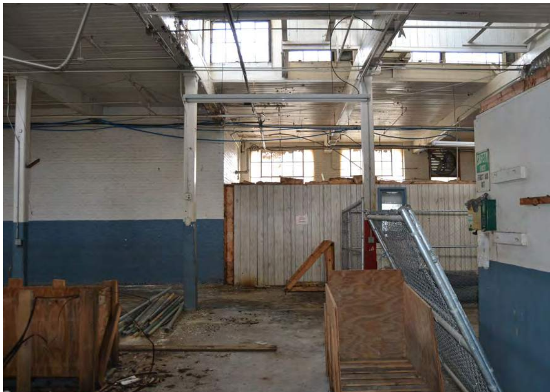
78. Grey Mill, 1926 Addition, Drying Room, Looking East
