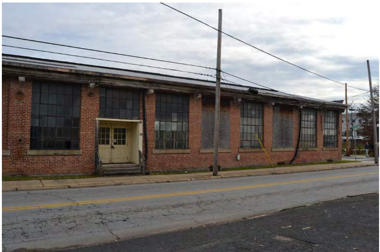
8. Grey Mill, 1915 Building, West Elevation, Looking Southeast
