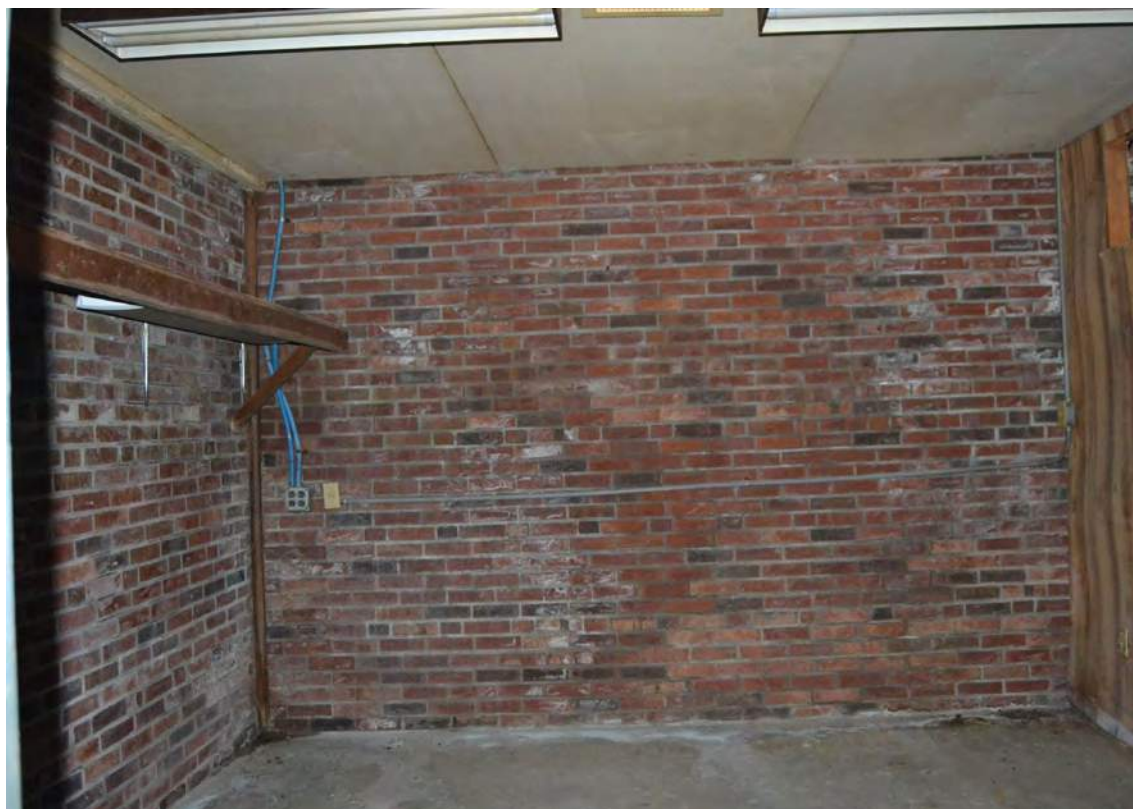
89. Grey Mill, 1970s Warehouse, Looking East
