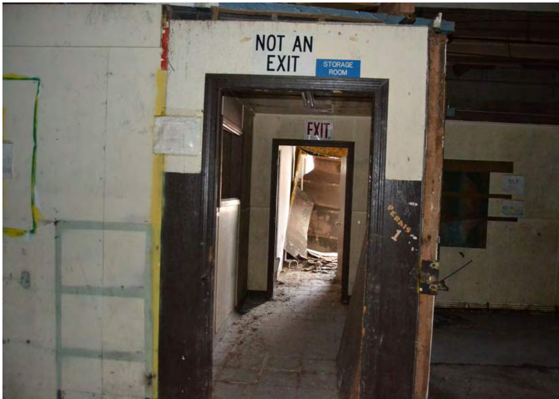
50. Grey Mill, 1947 Addition, Looking North
