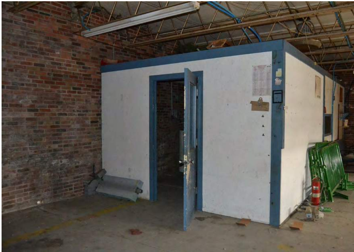
88. Grey Mill, 1970s Warehouse, Looking Northeast
