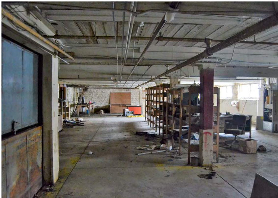
107. Grey Mill, Shipping and Storage Basement, Looking East
