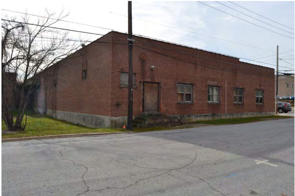
13. Grey Mill, 1947 Addition, North Elevation, Looking Southwest
