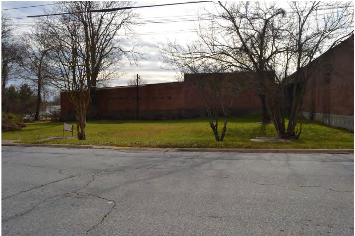
15. Grey Mill, 1947 Addition, North Elevation, Looking South
