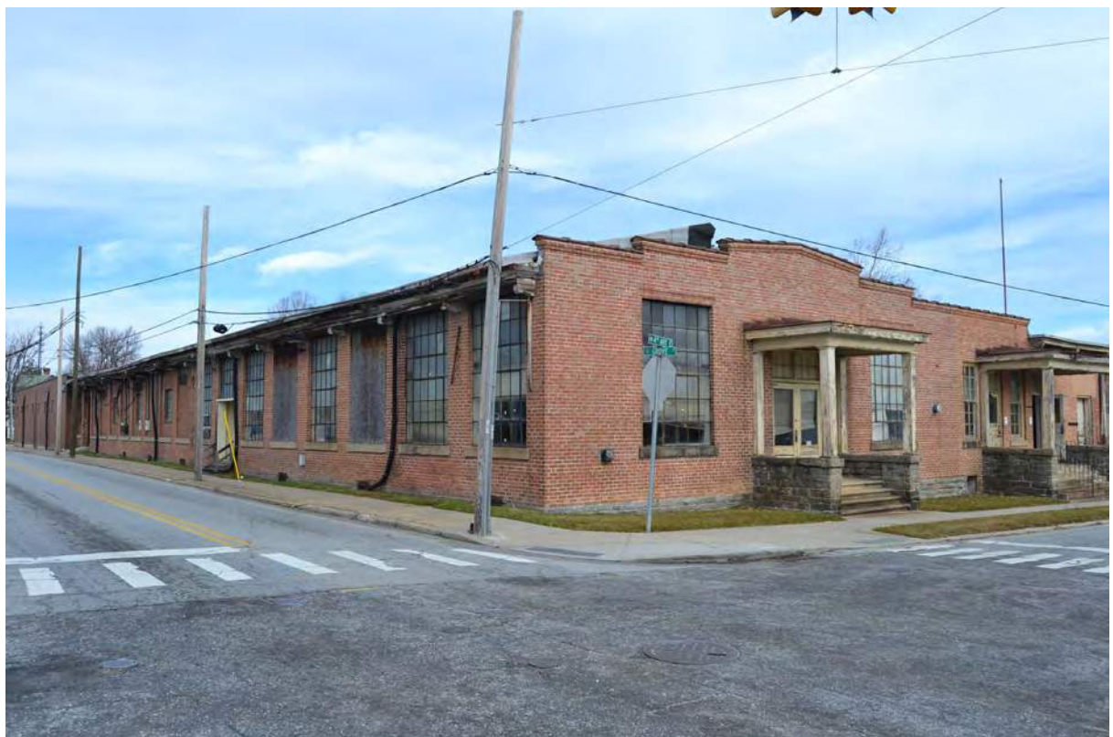
2. Grey Mill, 1915 Building, Southwest Corner, Looking Northeast
