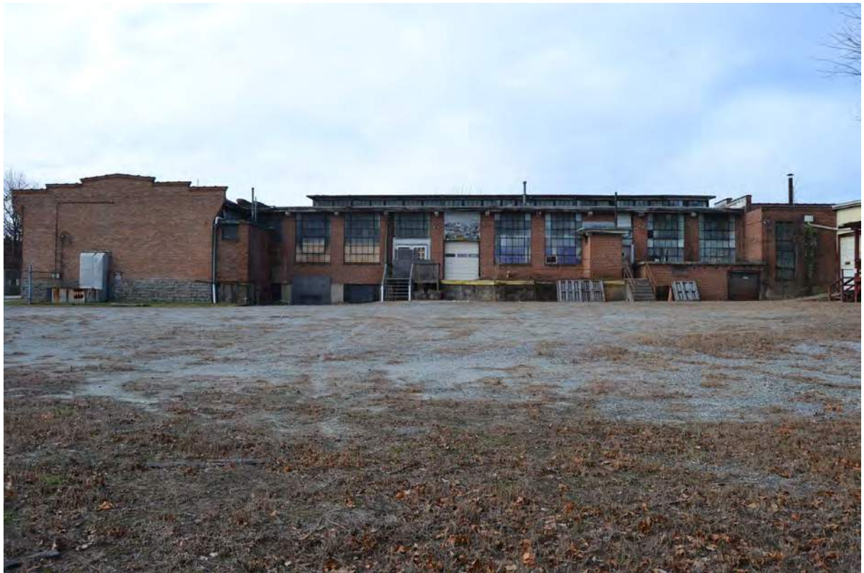
19. Grey Mill, 1919 Building, East Elevation, Looking West
