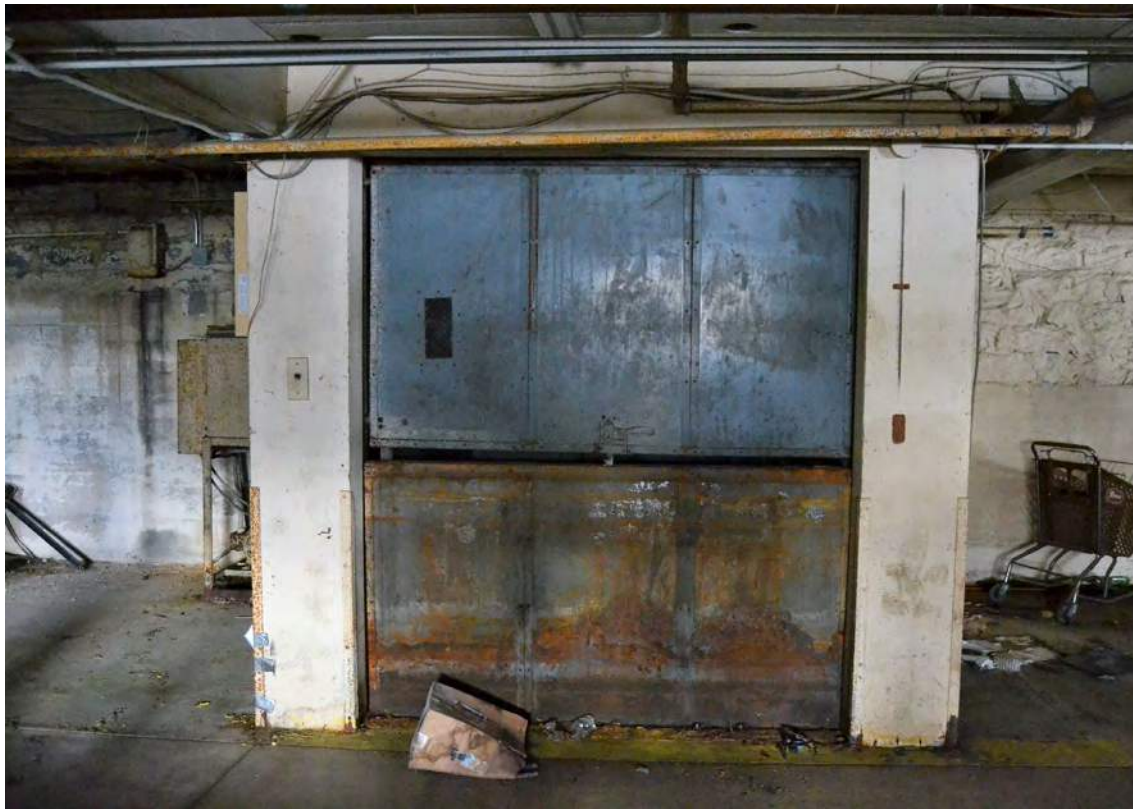
108. Grey Mill, Shipping and Storage Basement, Looking North
