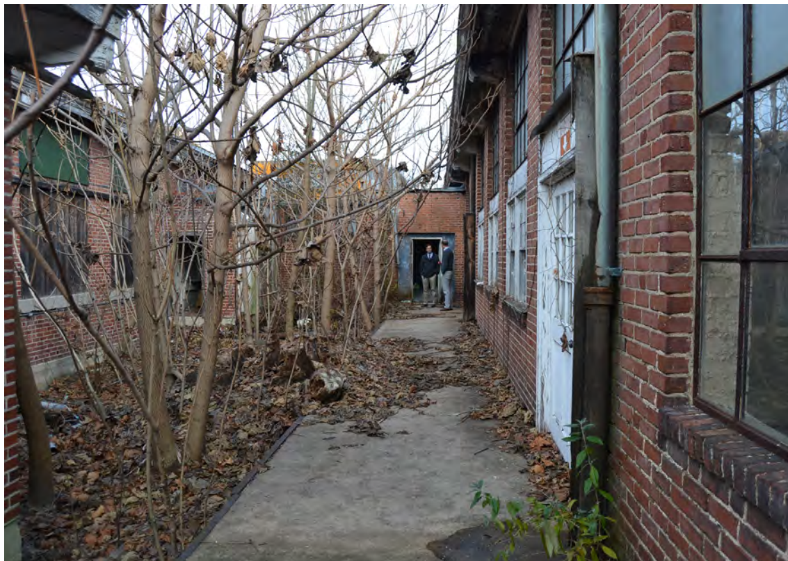
96. Grey Mill, Courtyard, Looking North
