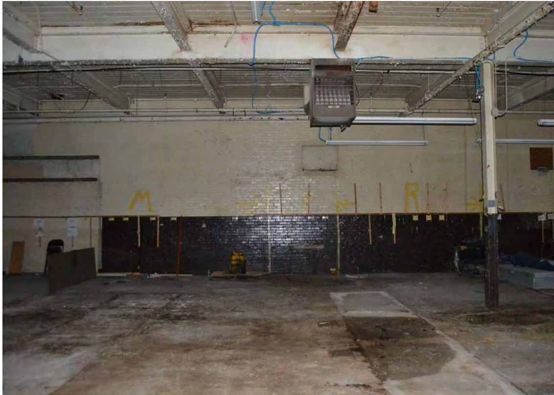
49. Grey Mill, 1947 Addition, Looking East
