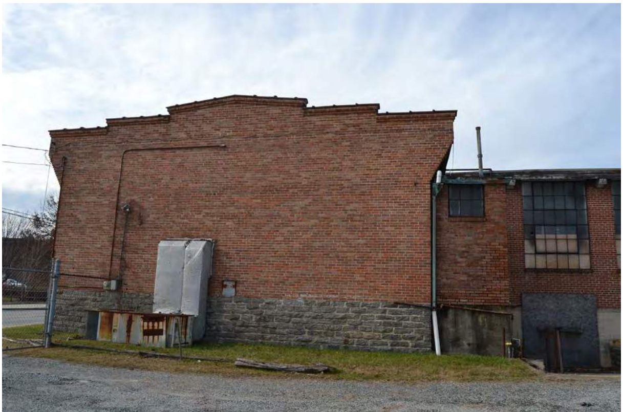
24. Grey Mill, 1919 Building, East Elevation, Looking West
