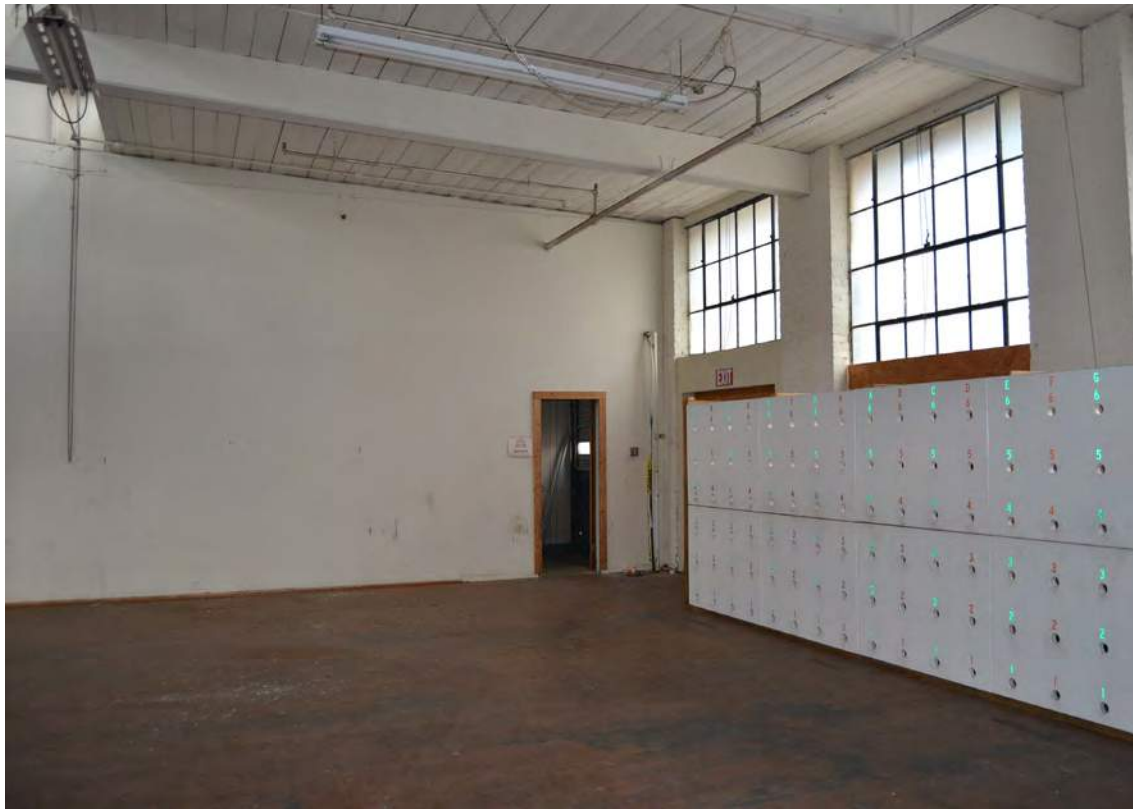
67. Grey Mill, 1926 Addition, Finishing Room, Looking Northeast
