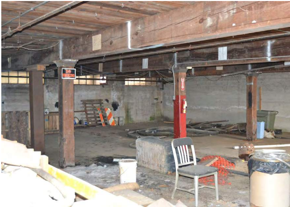
116. Grey Mill, Dye House Basement, Looking Northwest
