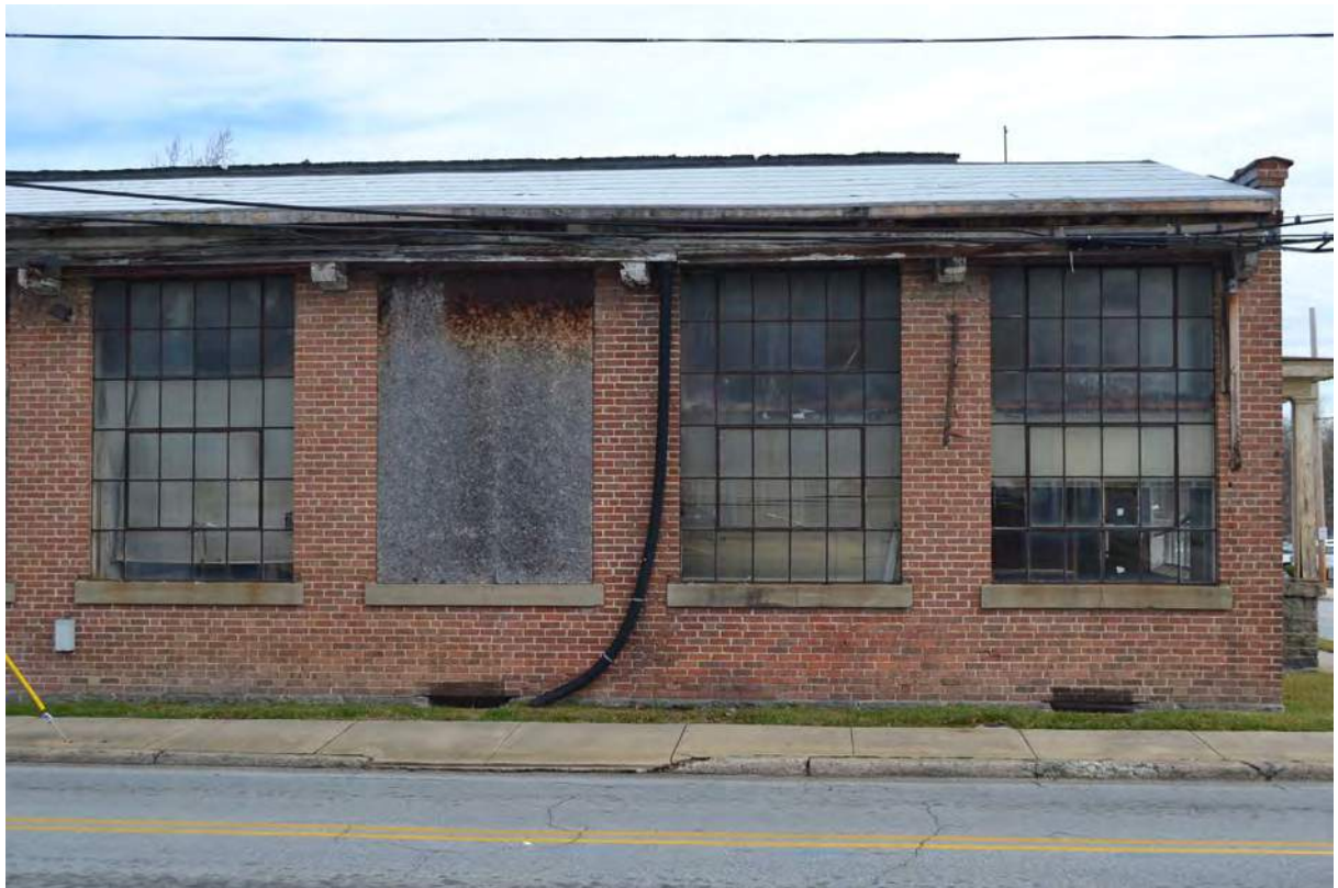
7. Grey Mill, 1915 Building, West Elevation, Window Detail
