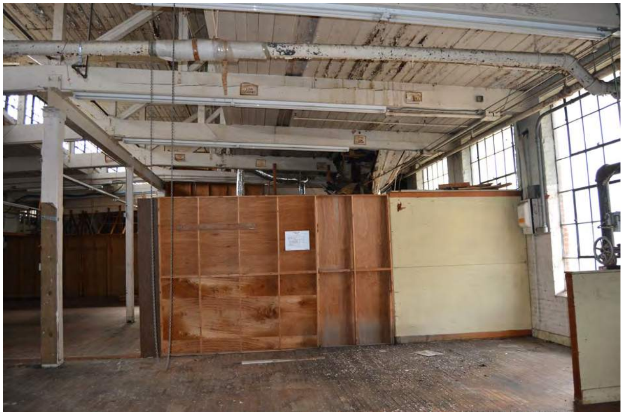
42. Grey Mill, 1915 Building, Looking South
