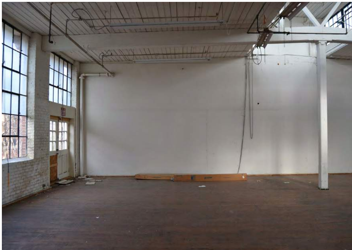
68. Grey Mill, 1926 Addition, Finishing Room, Looking North
