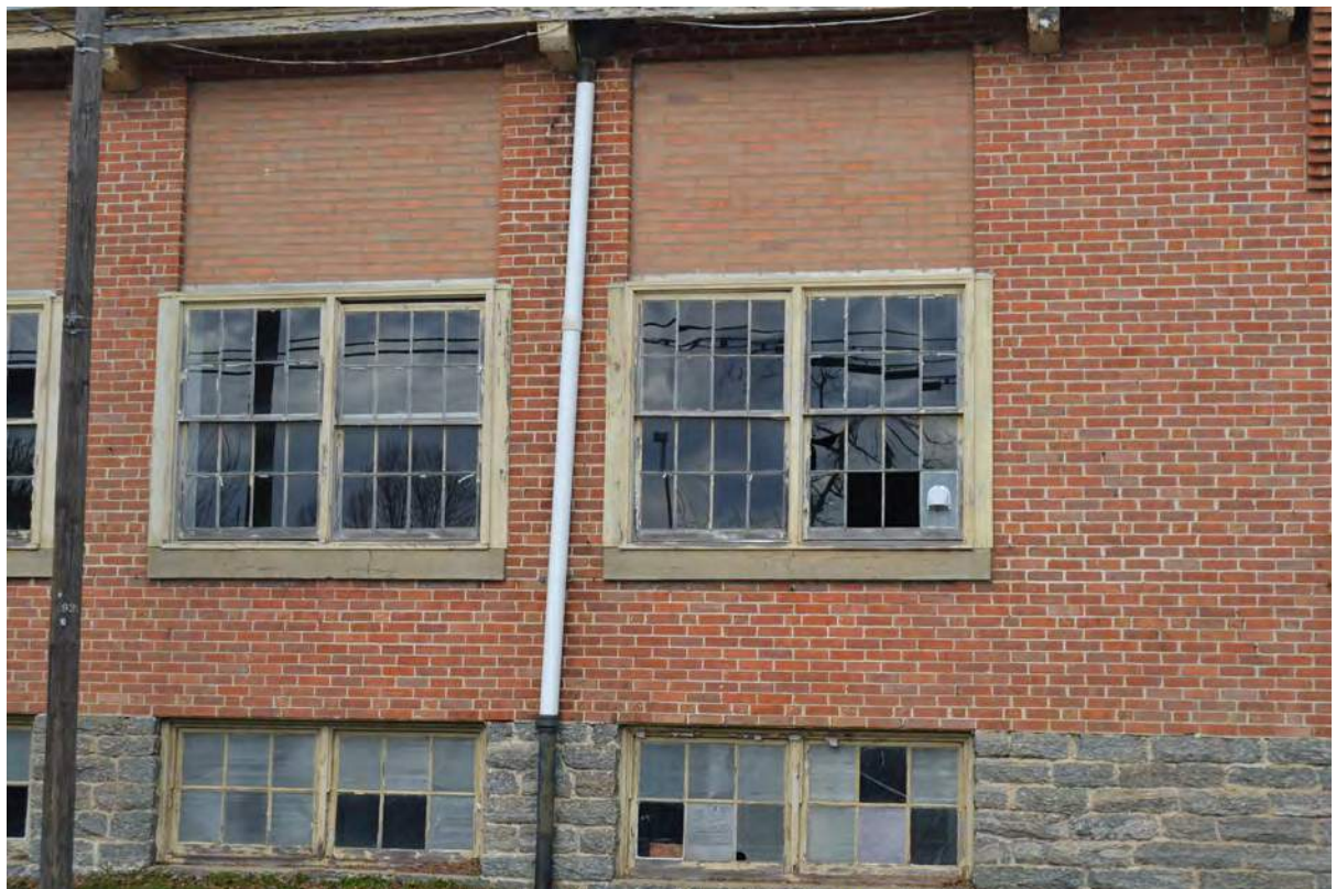
6. Grey Mill, 1919 Building, South Facade, Looking North
