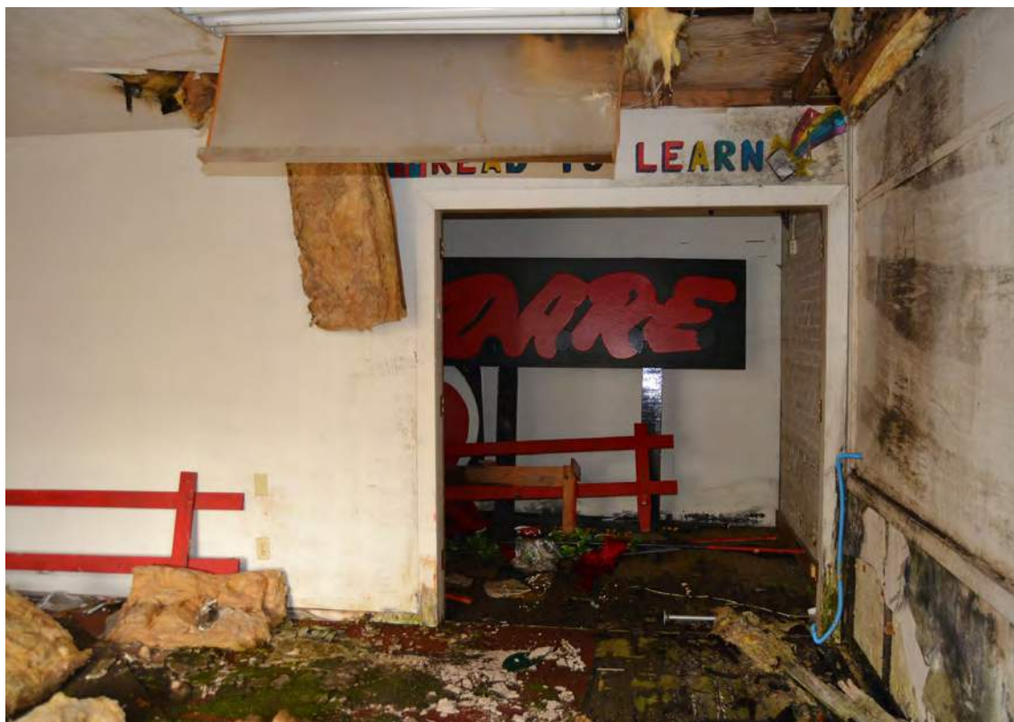
32. Grey Mill, 1915 Building, South End, Looking North
