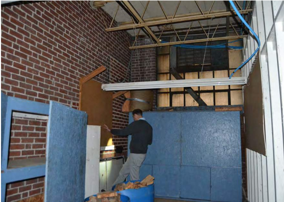
90. Grey Mill, 1970s Warehouse, Looking West
