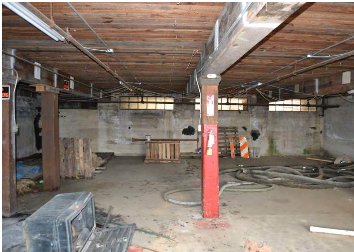
117. Grey Mill, Dye House Basement, Looking West
