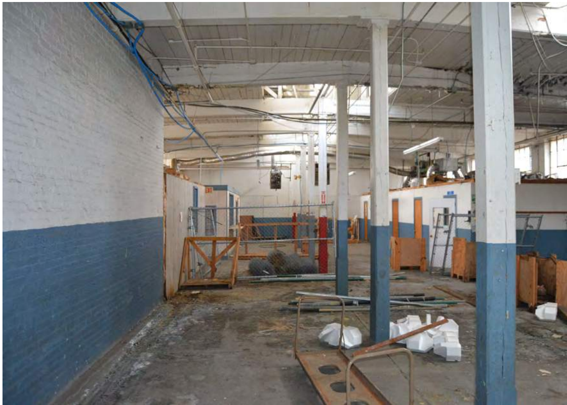
82. Grey Mill, 1926 Addition, Looking South
