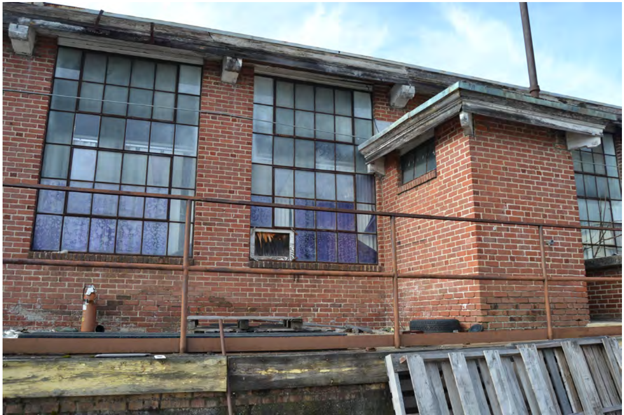
21. Grey Mill, 1919 Building, East Elevation, Window Detail
