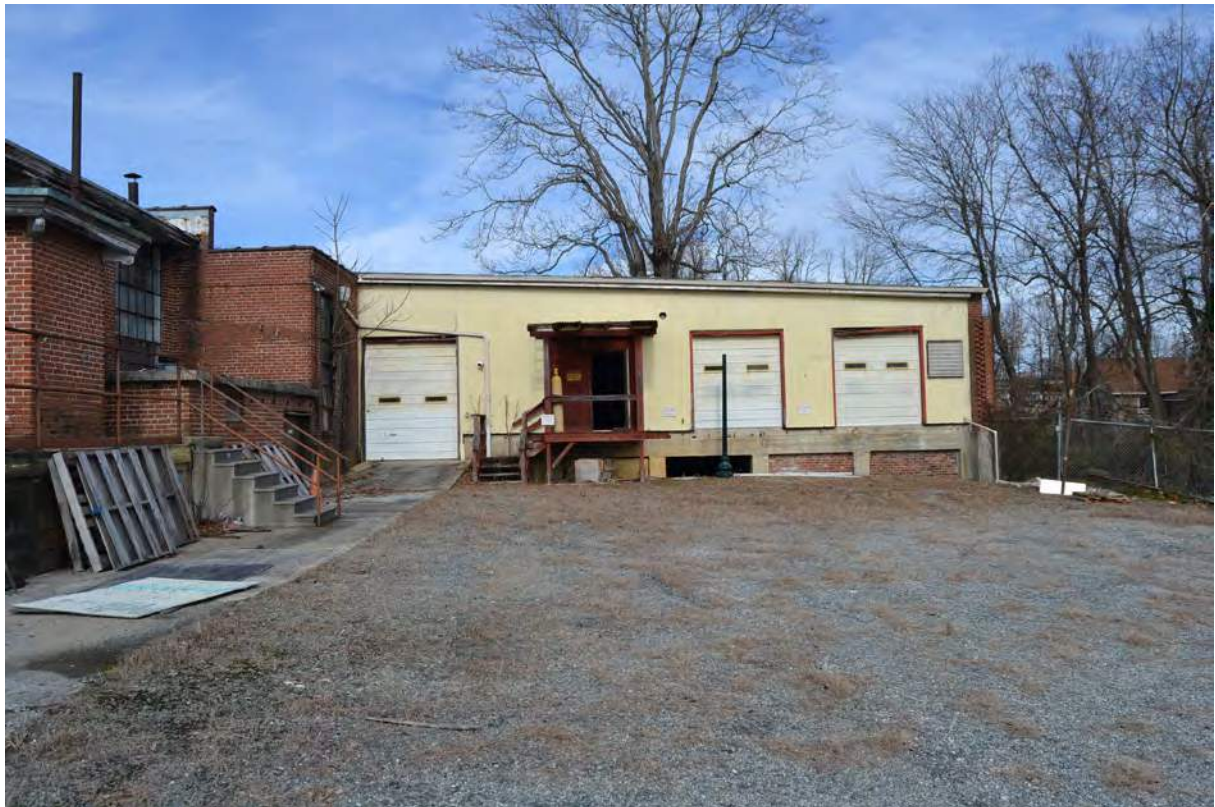
17. Grey Mill, 1970s Warehouse, Looking North
