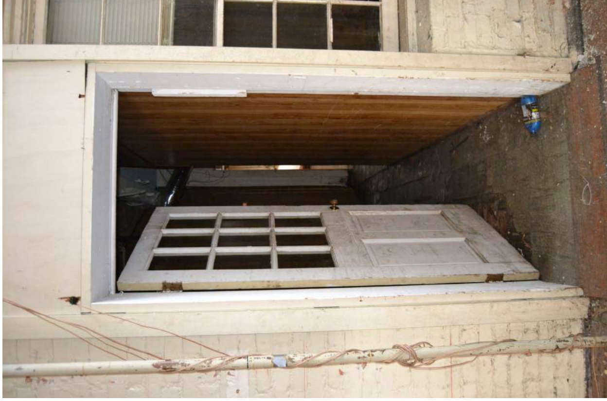
28. Grey Mill, Rear Office, Looking West
