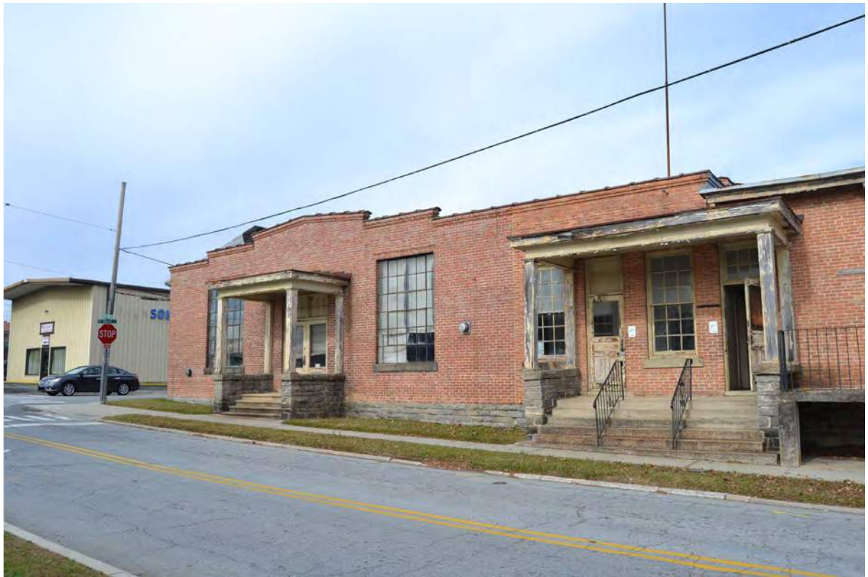
3. Grey Mill, 1915 Building, South Facade, Looking Northwest
