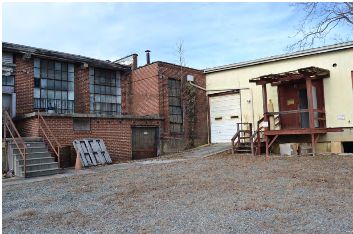
18. Grey Mill, 1919 Building and 1970s Warehouse, East Elevation, Looking Northwest
