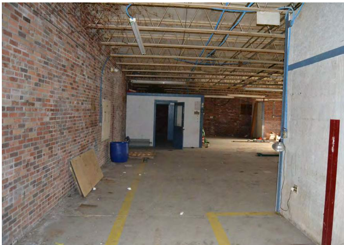
87. Grey Mill, 1970s Warehouse, Looking East
