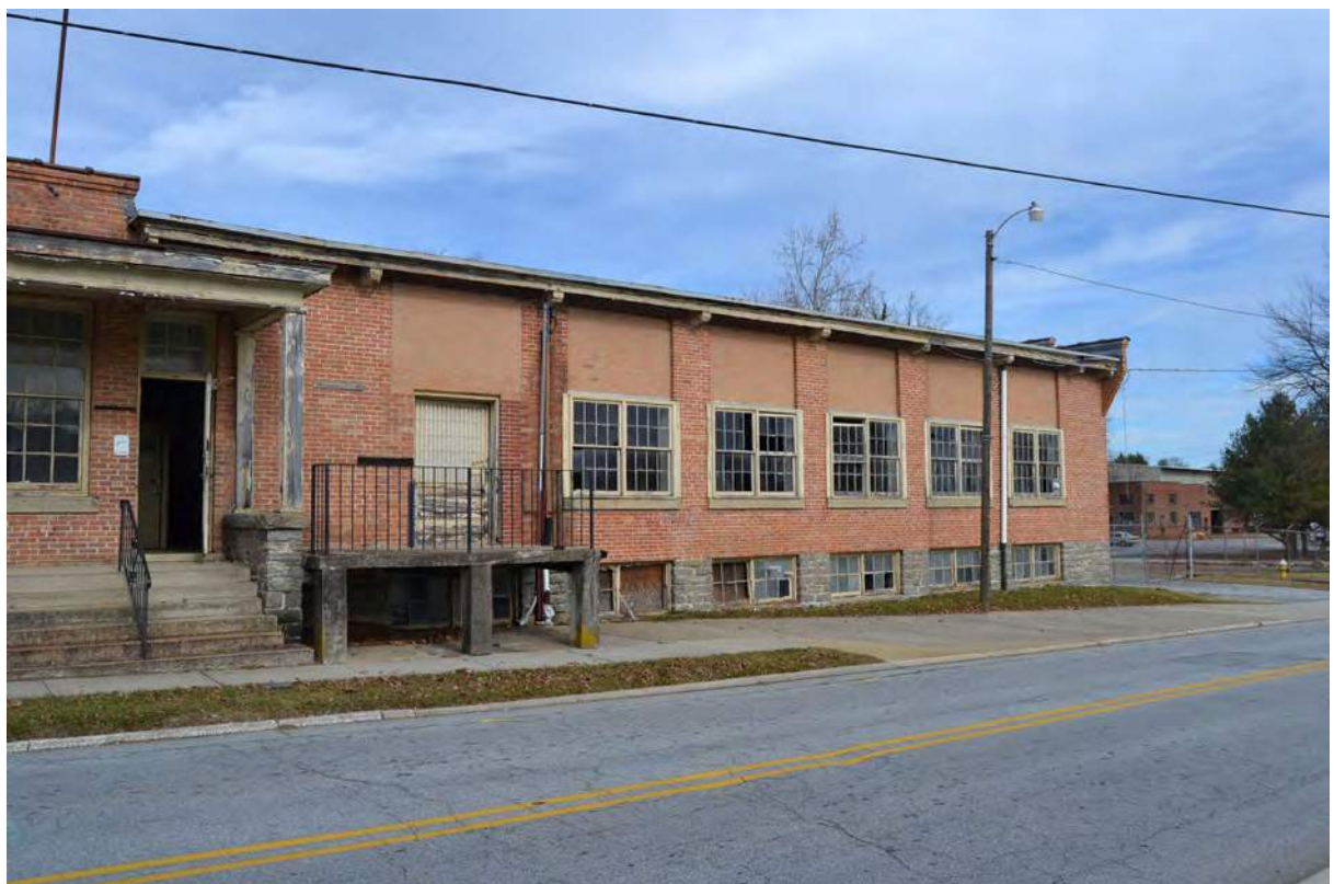
4. Grey Mill, 1919 Building, South Facade, Looking Northeast
