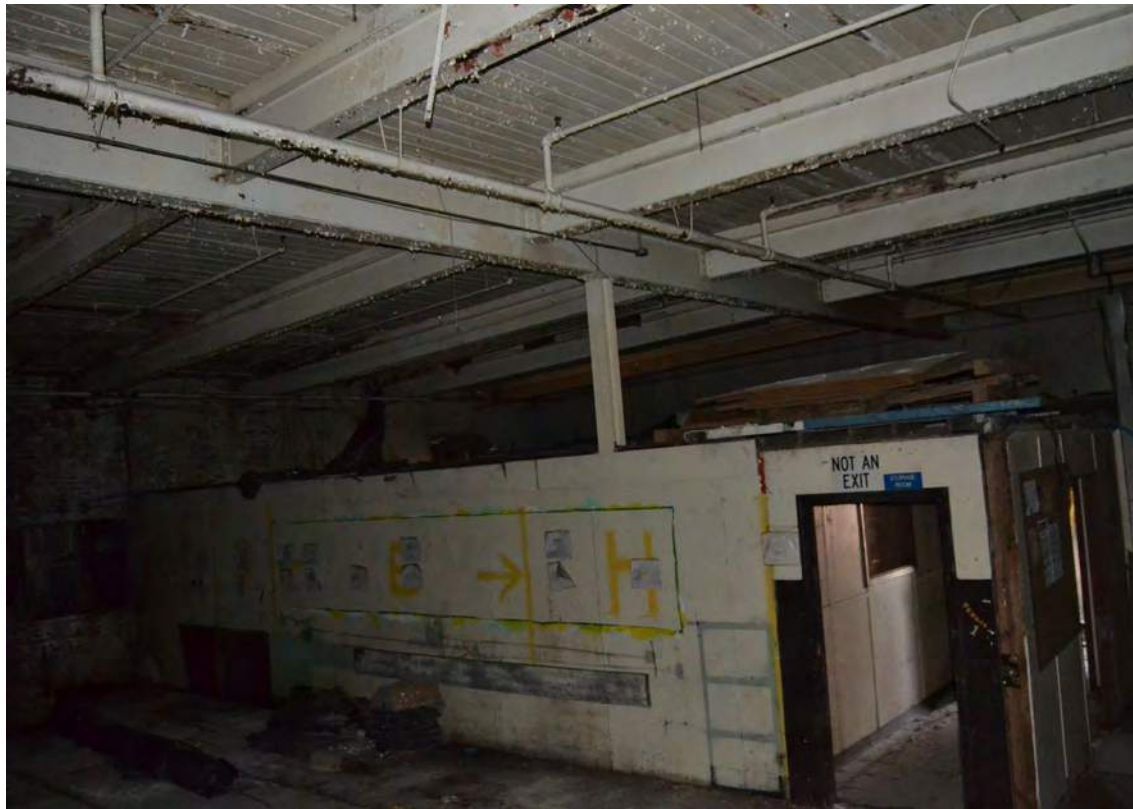
51. Grey Mill, 1947 Addition, Looking Northwest
