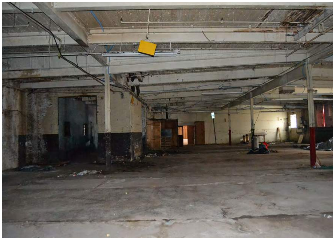
52. Grey Mill, 1947 Addition, Looking South
