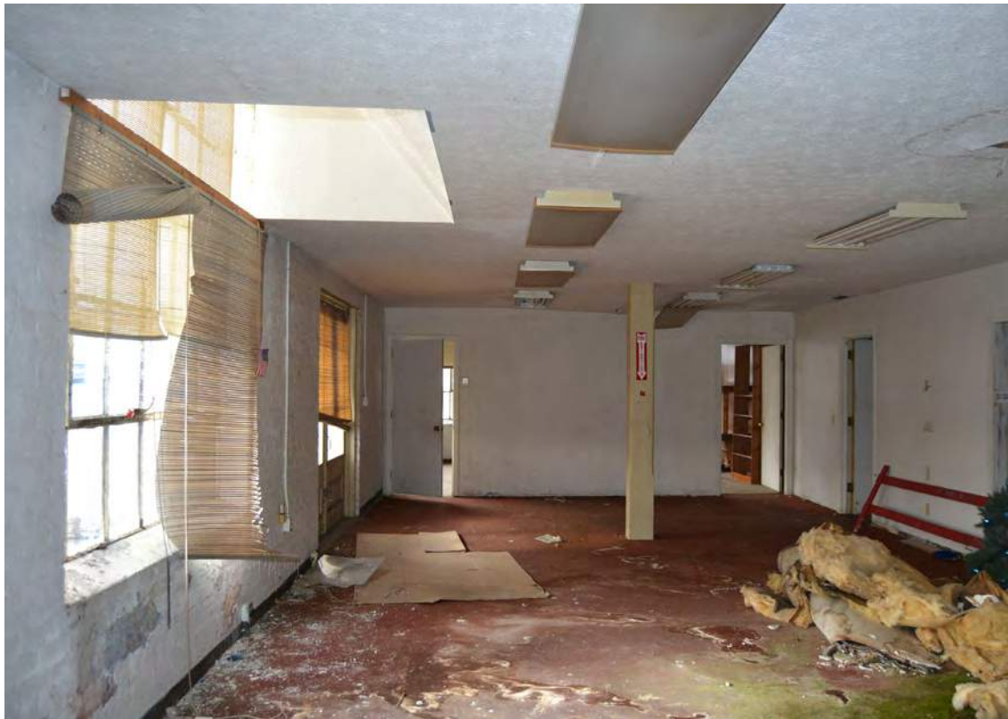
31. Grey Mill, 1915 Building, South End, Looking West
