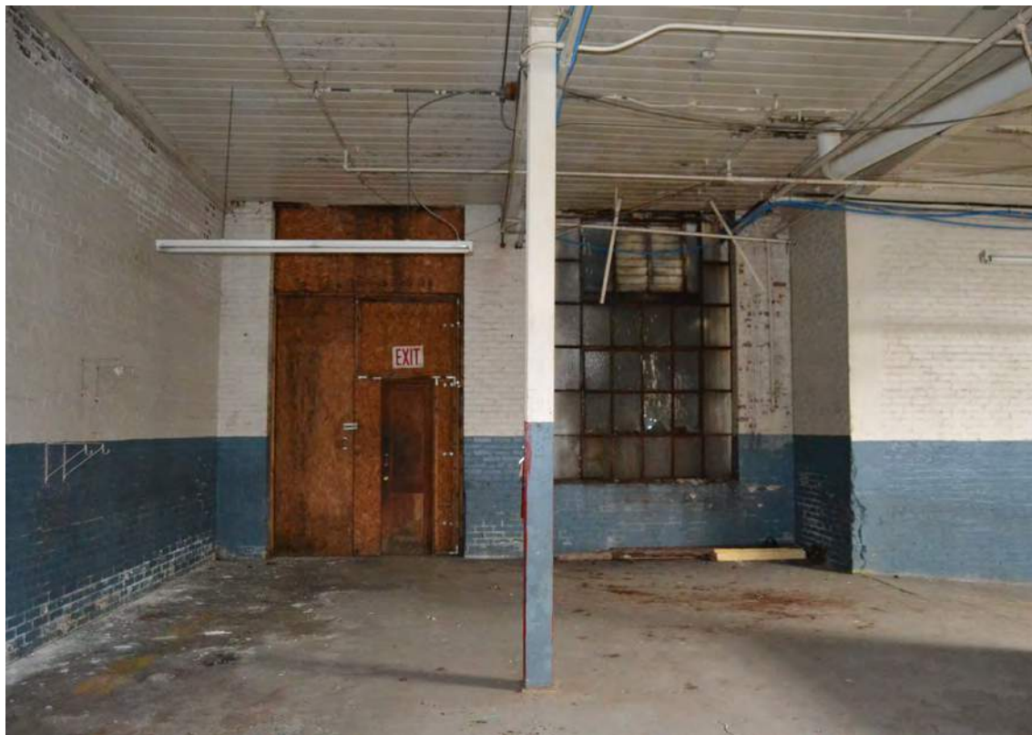
81. Grey Mill, 1926 Addition, Looking East
