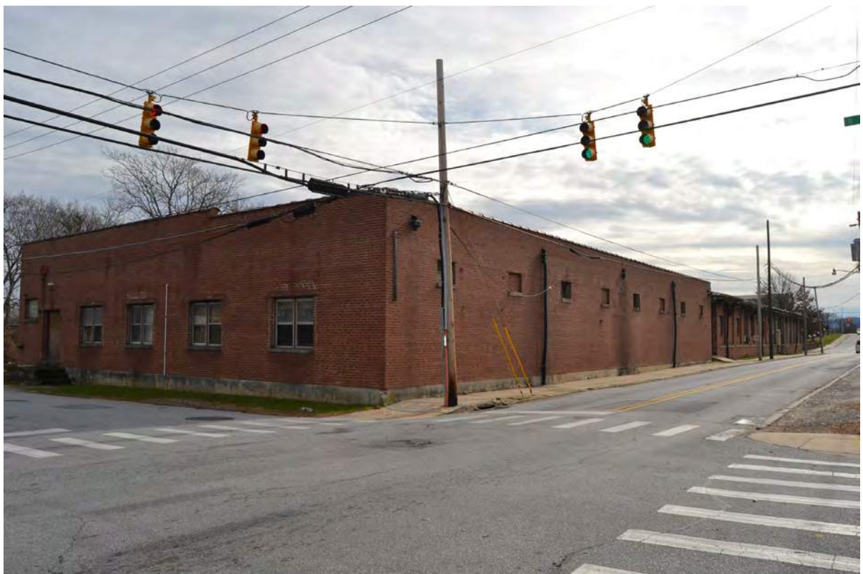
12. Grey Mill, 1947 Addition, Northwest Corner, Looking Southeast
