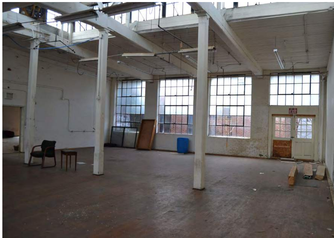
70. Grey Mill, 1926 Addition, Finishing Room, Looking Southwest
