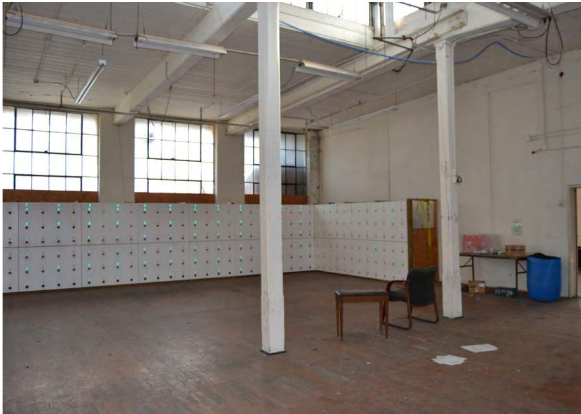
69. Grey Mill, 1926 Addition, Finishing Room, Looking Southeast
