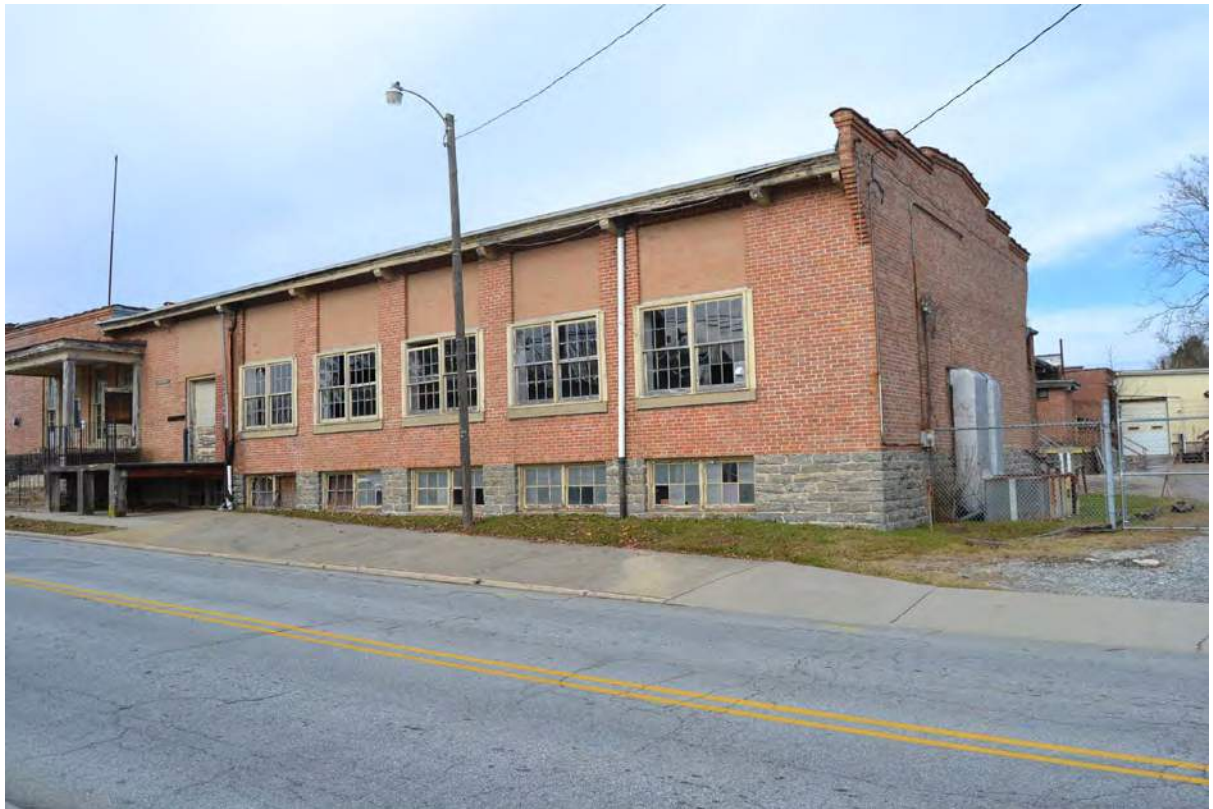
5. Grey Mill, 1919 Building, South Facade, Looking Northwest
