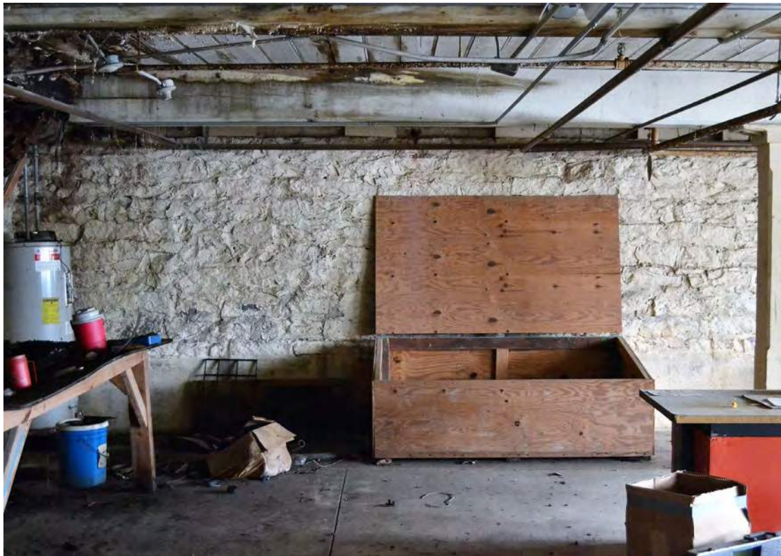
110. Grey Mill, Shipping and Storage Warehouse, Looking East
