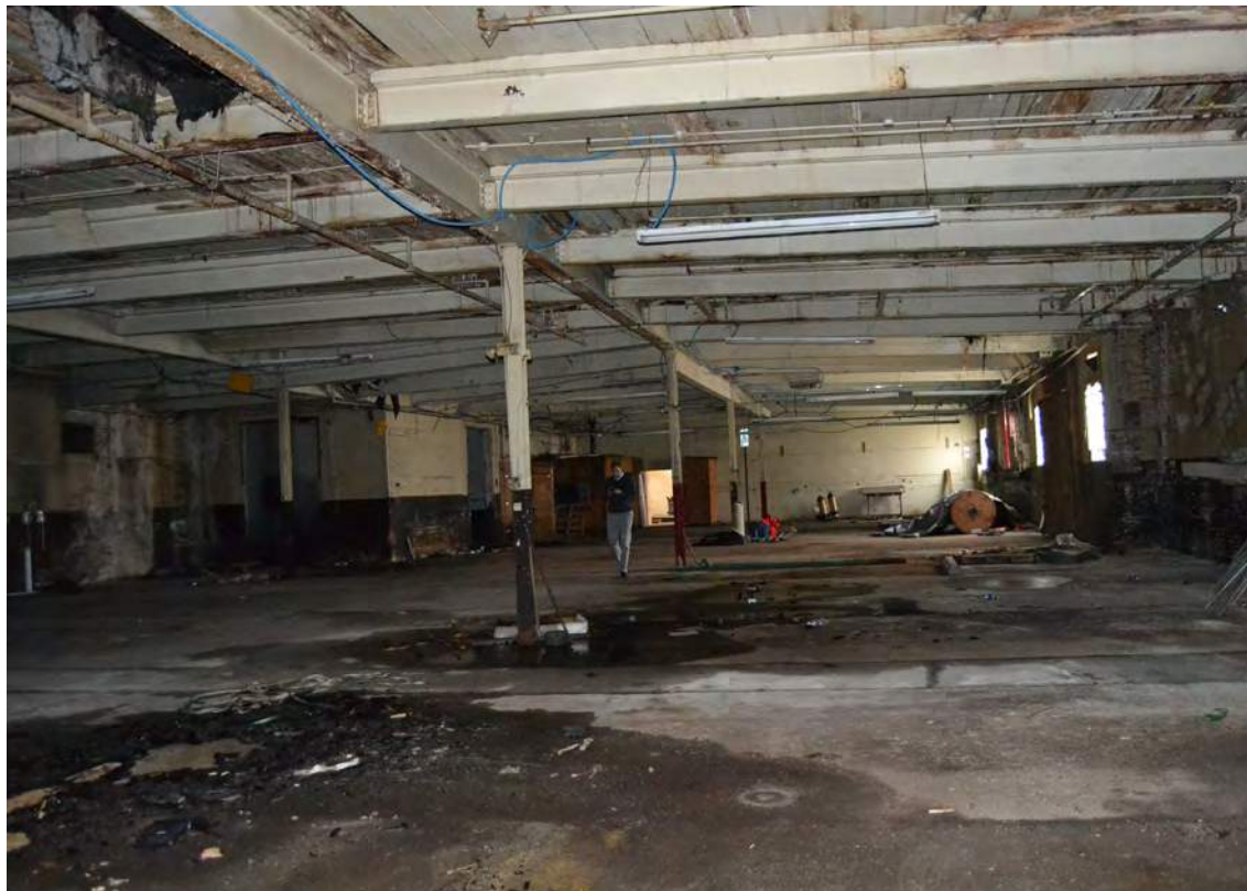
48. Grey Mill, 1947 Addition, Looking South
