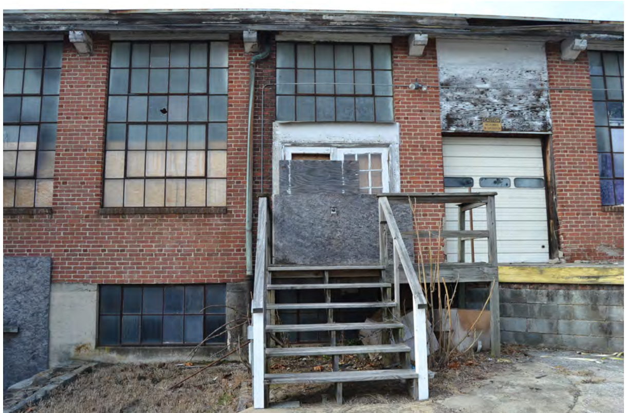
22. Grey Mill, 1919 Building, East Elevation, Loading Dock, Looking West
