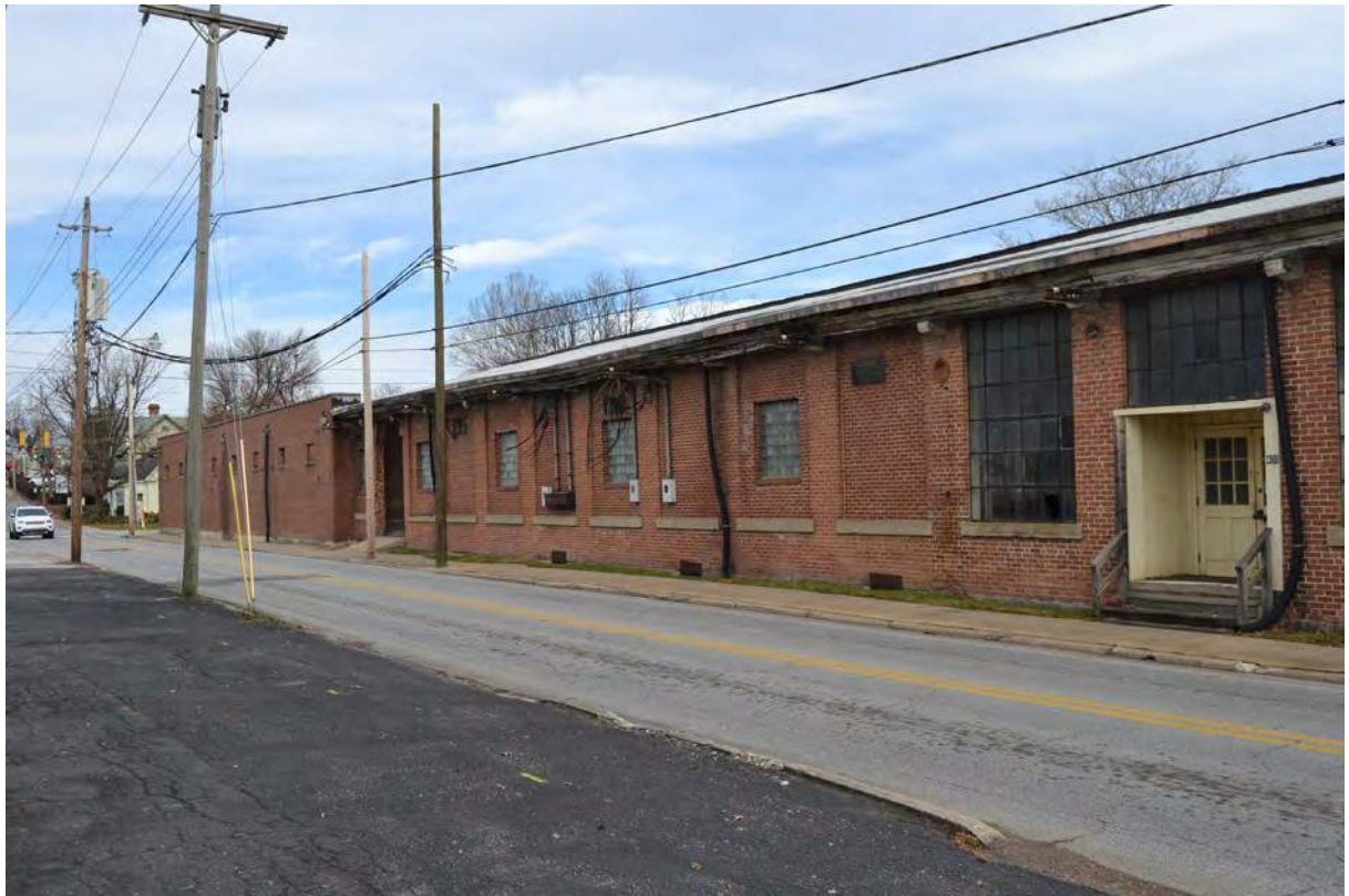
9. Grey Mill, 1915 Building, West Elevation, Looking Northeast
