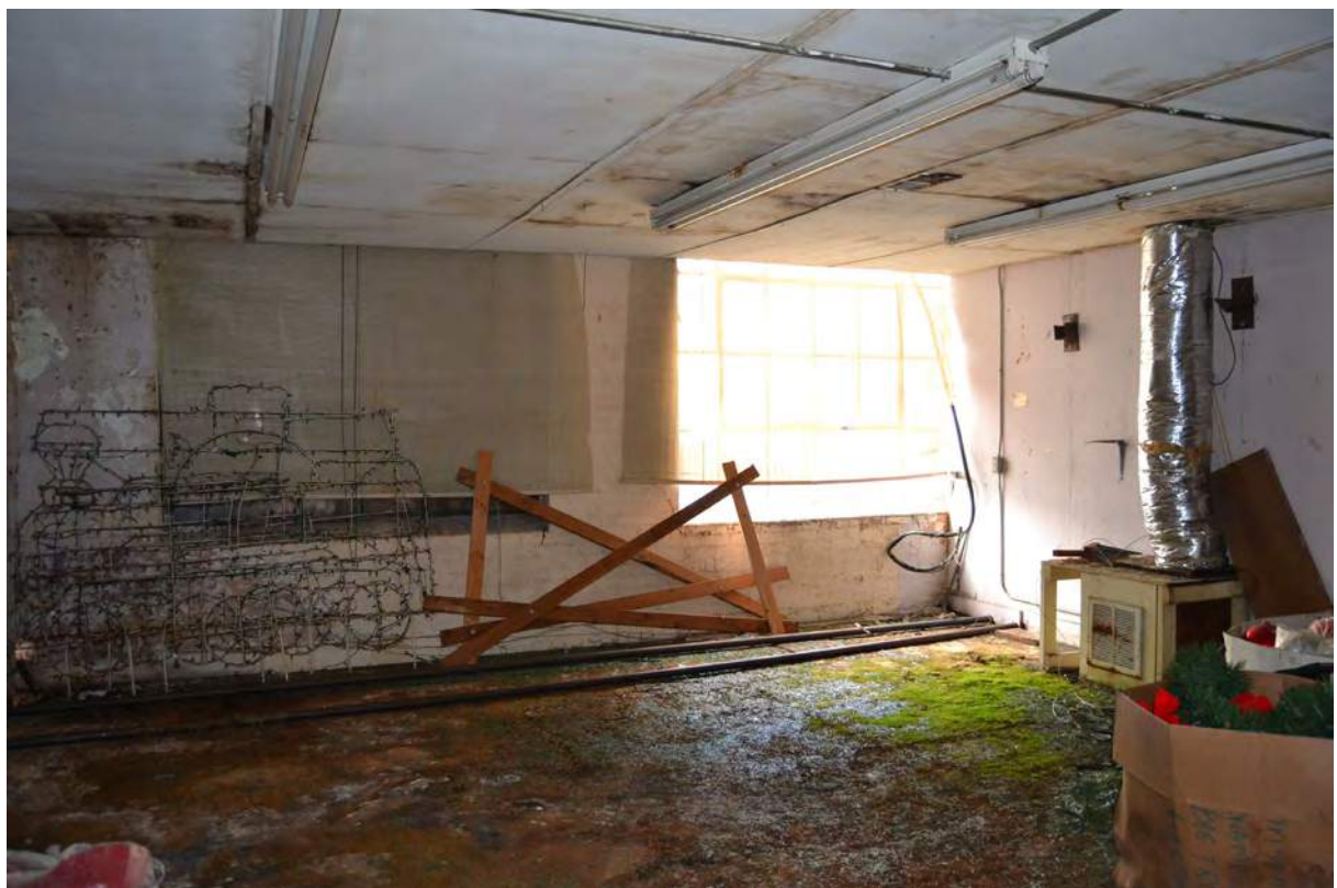
38. Grey Mill, 1915 Building, Looking West
