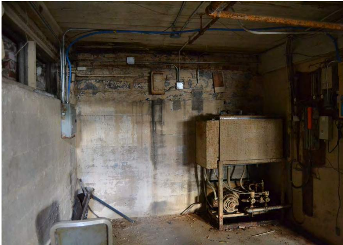
106. Grey Mill, Shipping and Storage Basement, Looking North
