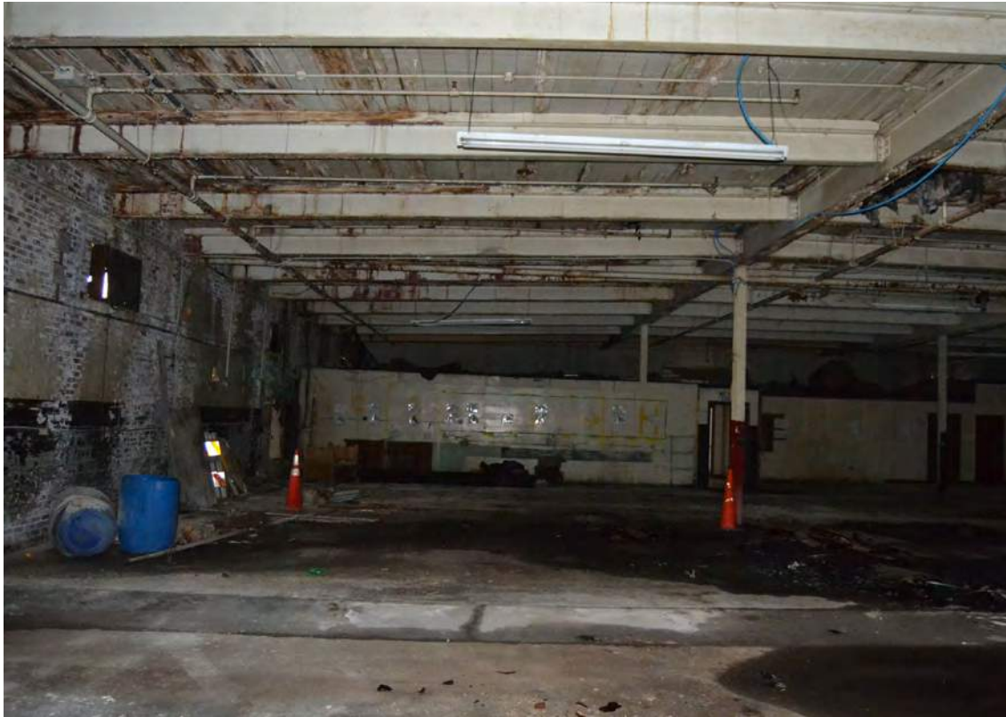
47. Grey Mill, 1947 Addition, Looking North
