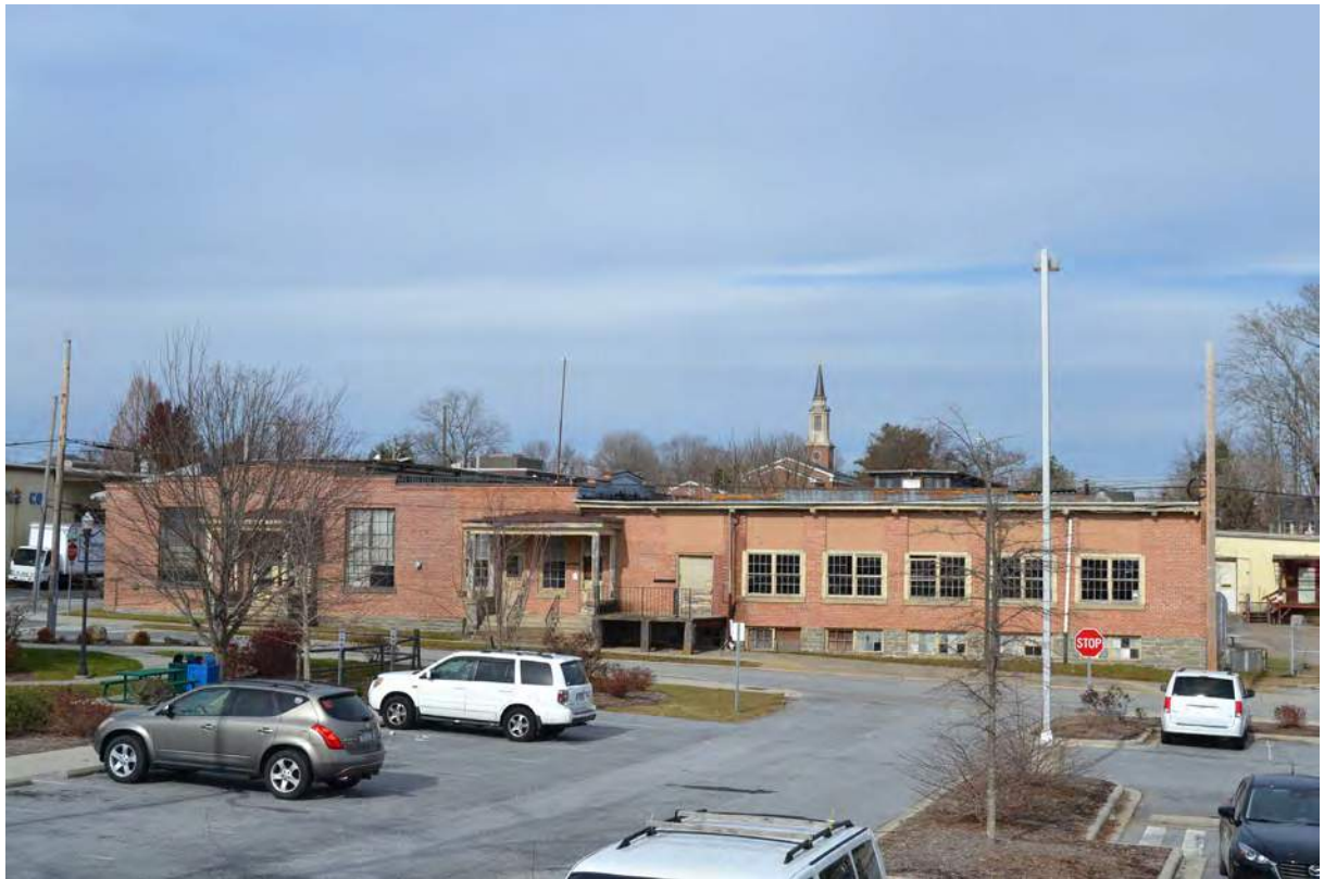
1. Grey Mill, South Facade, Looking North
