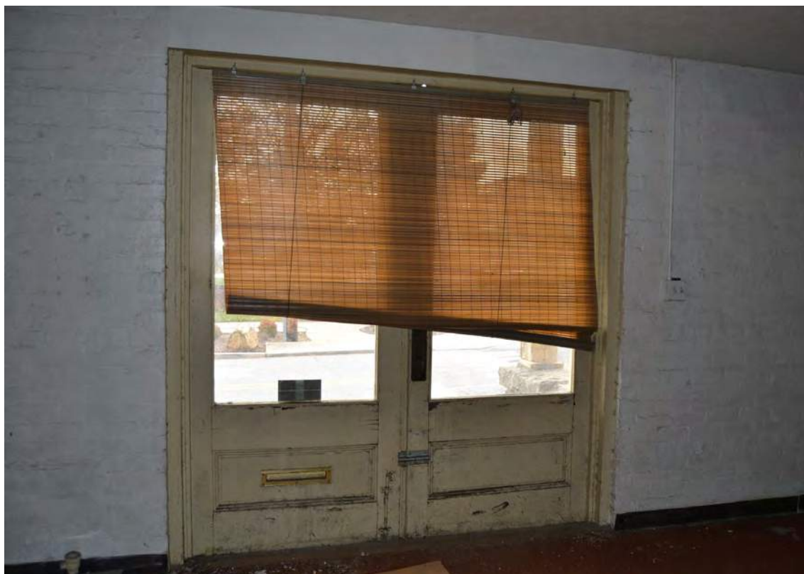
34. Grey Mill, 1915 Building Entrance Doors, Looking South
