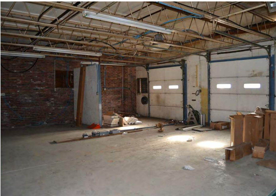
91. Grey Mill, 1970s Warehouse, Looking Southeast
