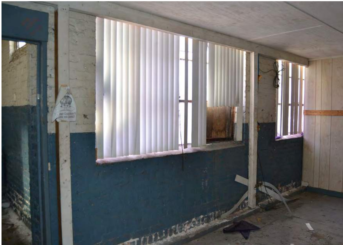
86. Grey Mill, 1926 Addition, Looking Southeast
