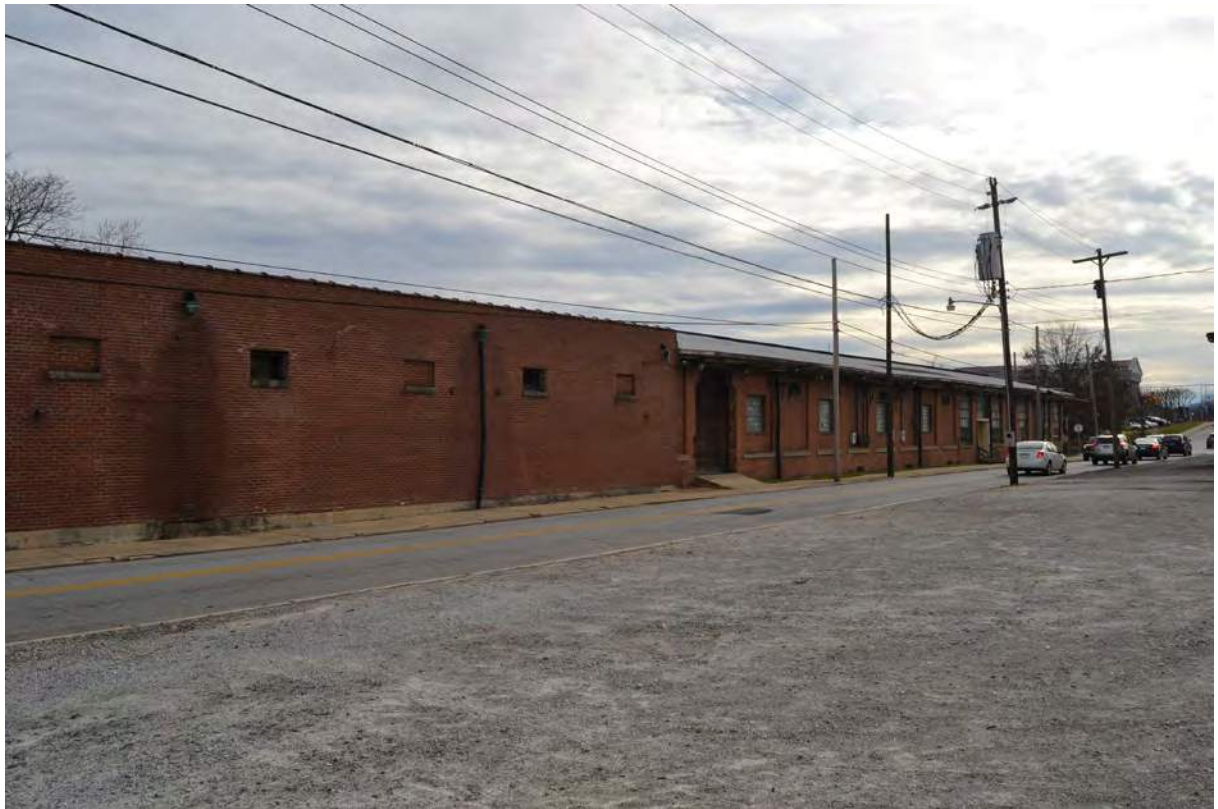
11. Grey Mill, 1947 Addition and 1915 Building, West Elevation, Looking Southeast
