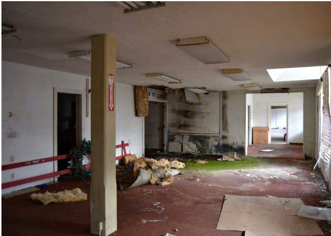
33. Grey Mill, 1915 Building, South End, Looking East
