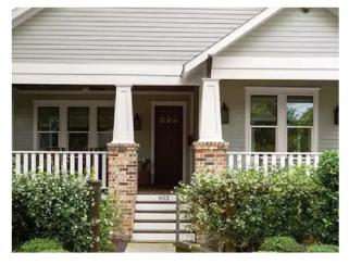
HERE'S AN EXAMPLE OF BRICK WING WALLS & WOODEN STEPS ON A CRAFTSMAN STYLE HOME. DOING WOOD FOR STEPS TOOK OUR COST OF THE REPAIR FROM JUST UNDER 17K TO JUST OVER &K. DOING ALL BRICK IS COST PROHIBITIVE BUT STEPS ARE IN MAJOR NEED OF REPAIR BOTH AESTHETICALLY & FOR SAFETY.
