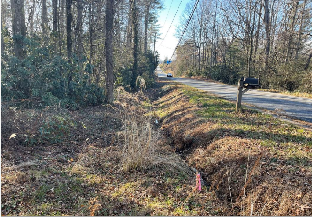
View of Waddell Drive frontage.
