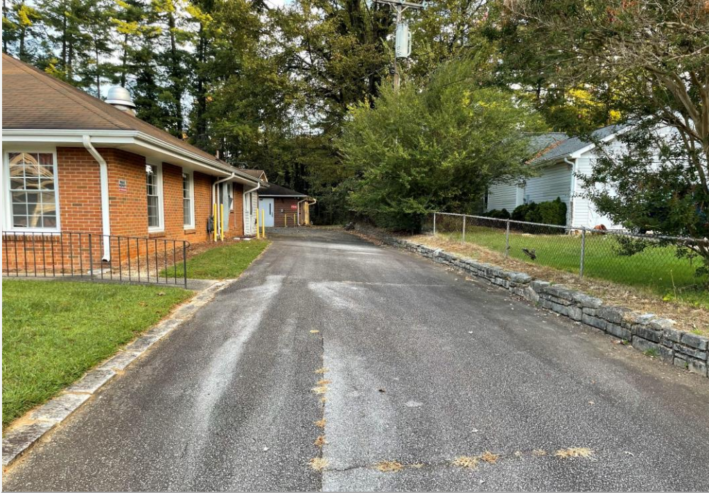
View of existing drive on the eastern property boundary proposed to remain.
