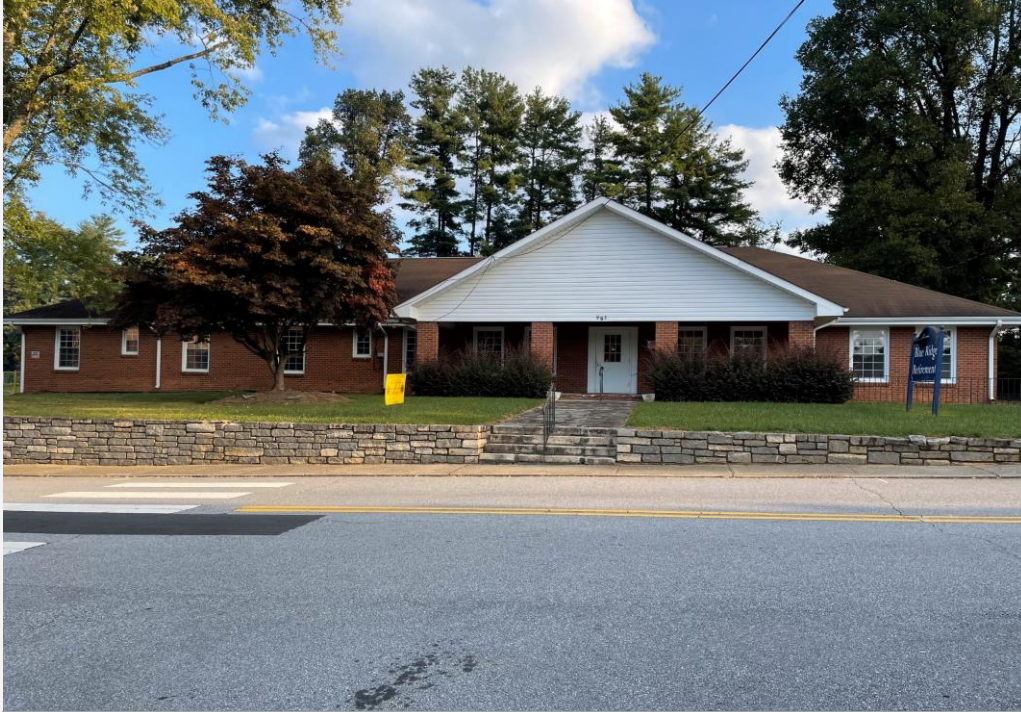
View of existing structure located at 913 9 th Ave. W. from the Hendersonville Middle School property to the south.
