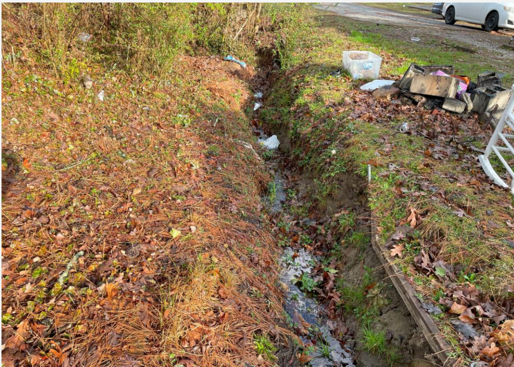
View of the area depicted as a blueline stream on the northeastern property boundary (after a rainfall event). Debris is from the adjacent property.
