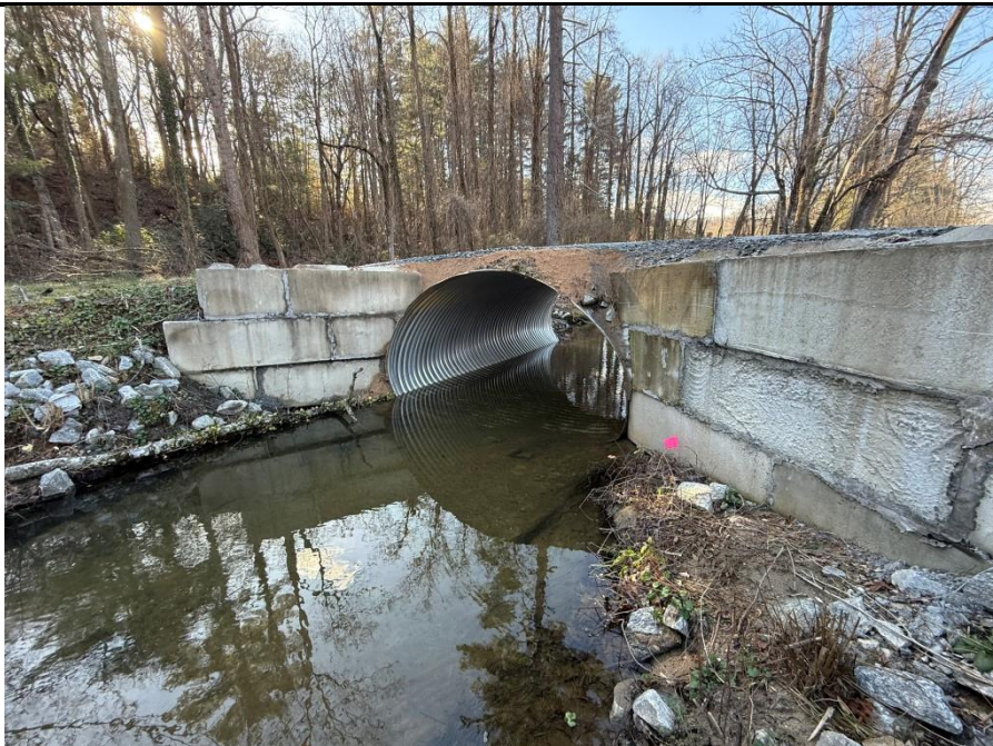
Photo 6: ST1 – culvert and bridge for driveway
