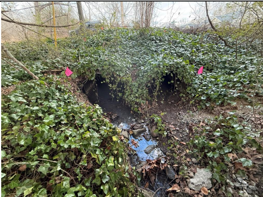
Photo 8: ST2 entering the property at Haywood Road via 2 metal culverts
