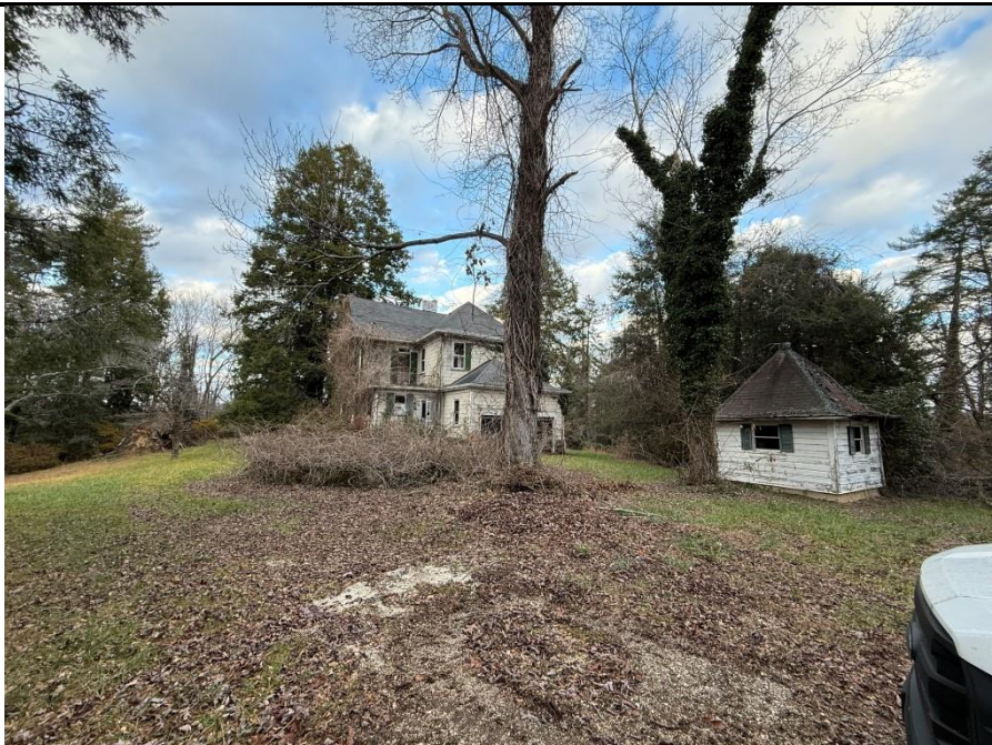
Photo 2: Subject property (southern portion, dilapidated structures).
