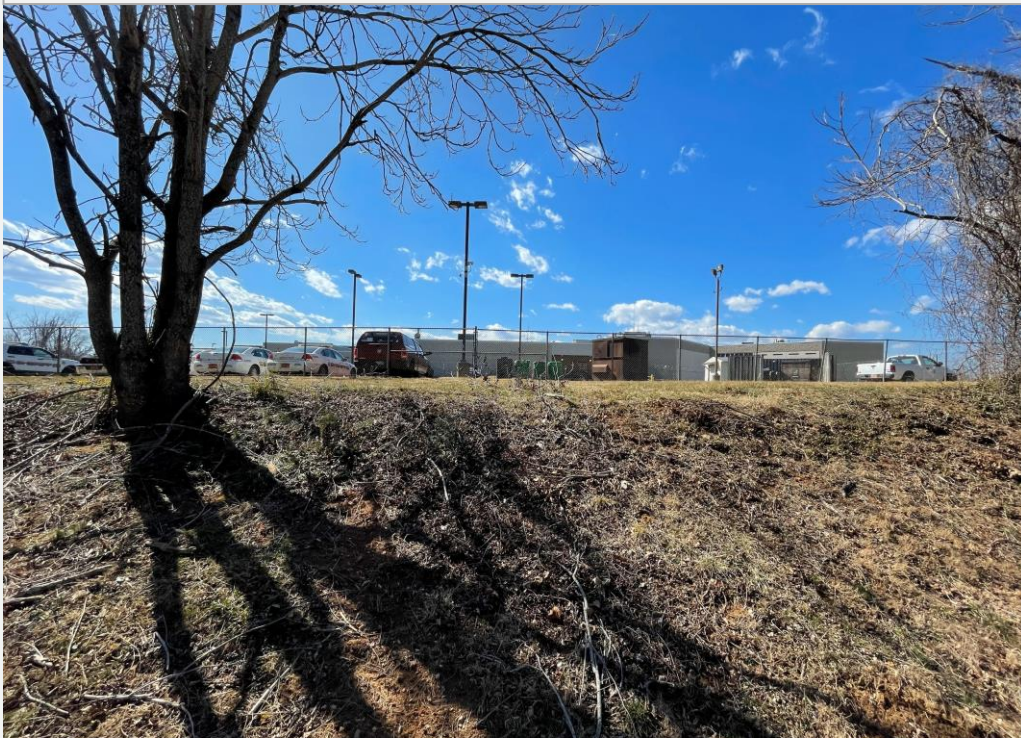
The rear of the existing detention center.
