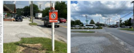
This project will need to include drainage and utility infrastructure adjustments, as well as driveway modifications and new ADA ramps.
