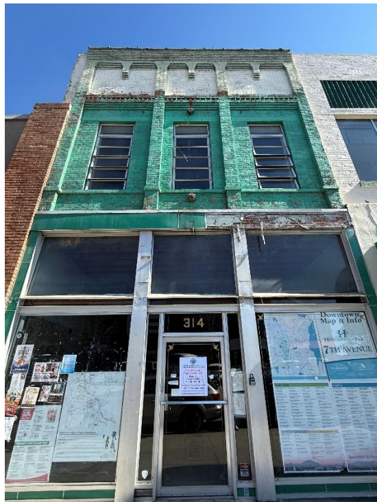
Close up photo of storefront facade
