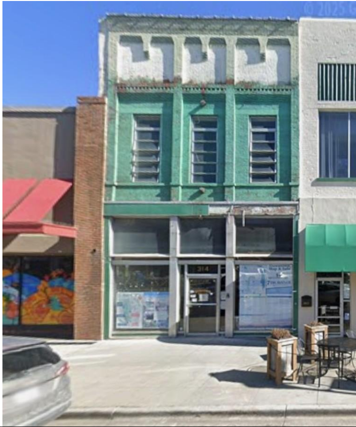
Existing front façade of 314 N Main Street.
