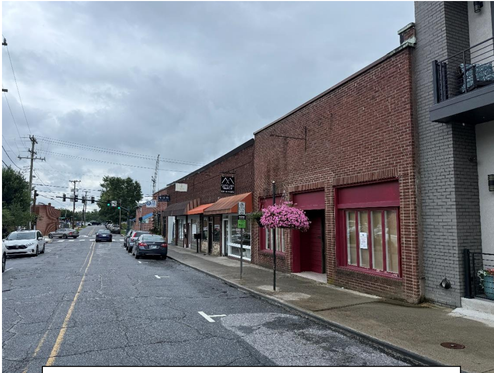
View of 3 rd Avenue looking east with subject property in foreground.
