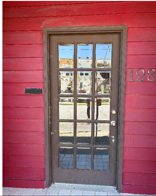
Non-original front door.
