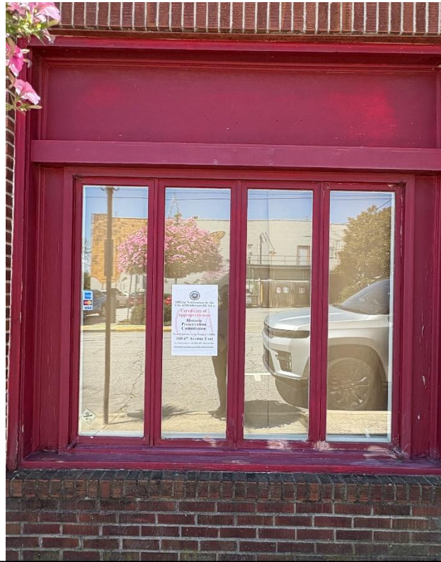
Westernmost infilled windows. Proposal will remove entire window and trim unit and replace with aluminum windows.
