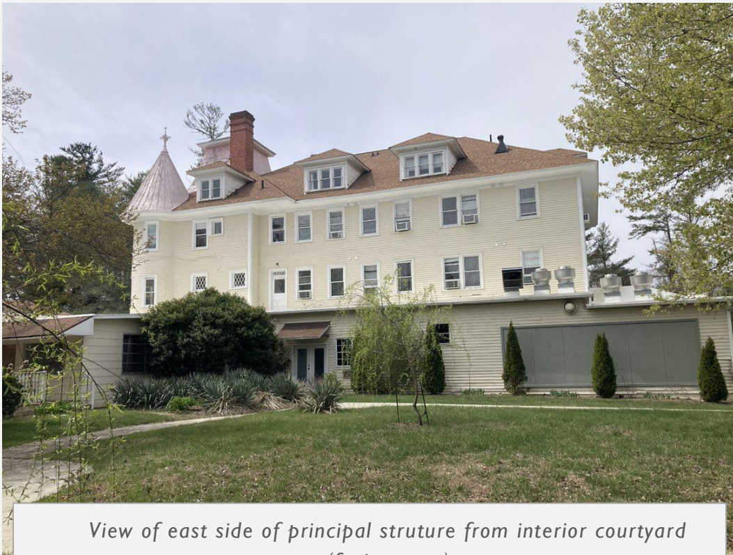
View of principal building at subject property (facing northeast)
