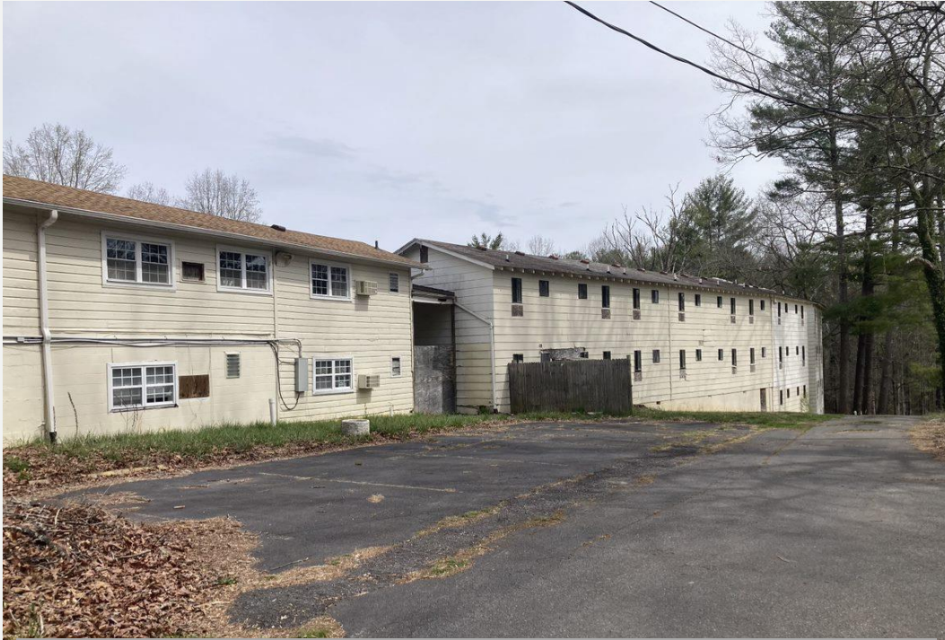
Facing north. View of rear of south wing and some existing parking
