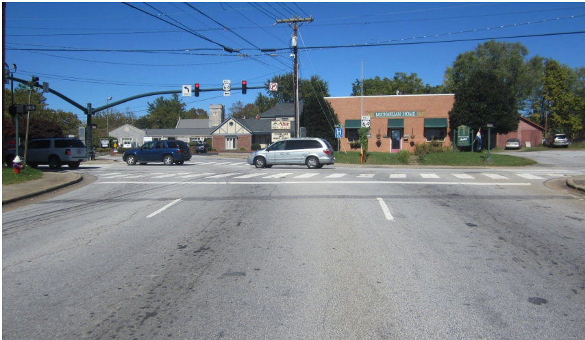
Photo of the intersection of 7th Avenue with King Street taken from the southern approach. The skewed intersection reduces sight distance for drivers turning left onto 7th Avenue, decreasing the visibility of pedestrians crossing the west leg.
