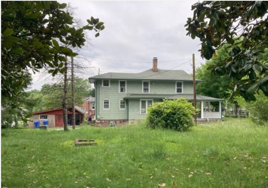
View of adjacent property to the west.
