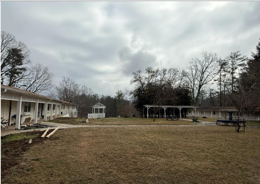
Center of property looking east. The building to the left will be adaptively reused as art studios.
