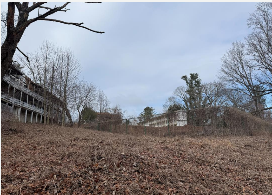
View from the easternmost part of the property looking west. The building to the left is proposed to be demolished.
