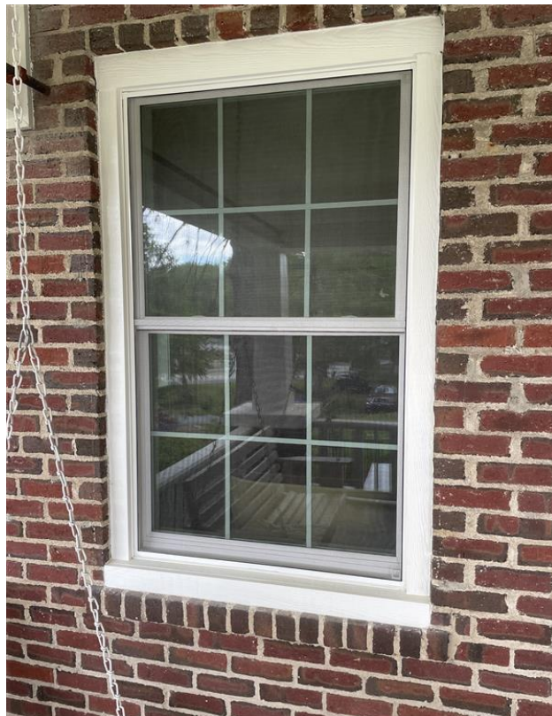
Windows located on front porch. Photo provided by Staff.
