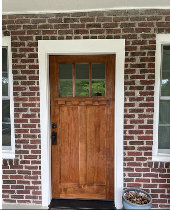
Replacement front door. Photo provided by Staff.
