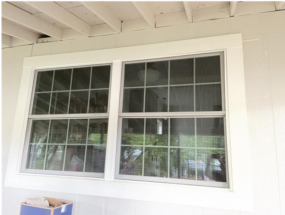
Windows located on southern façade of addition. Photo provided by Staff.
