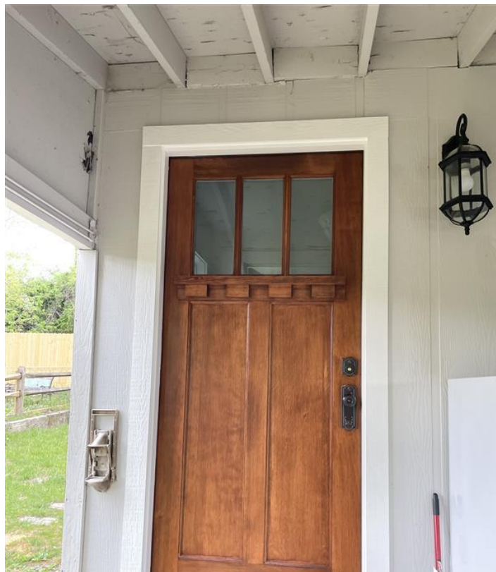
Door located on southern façade of addition. Photo provided by Staff.
