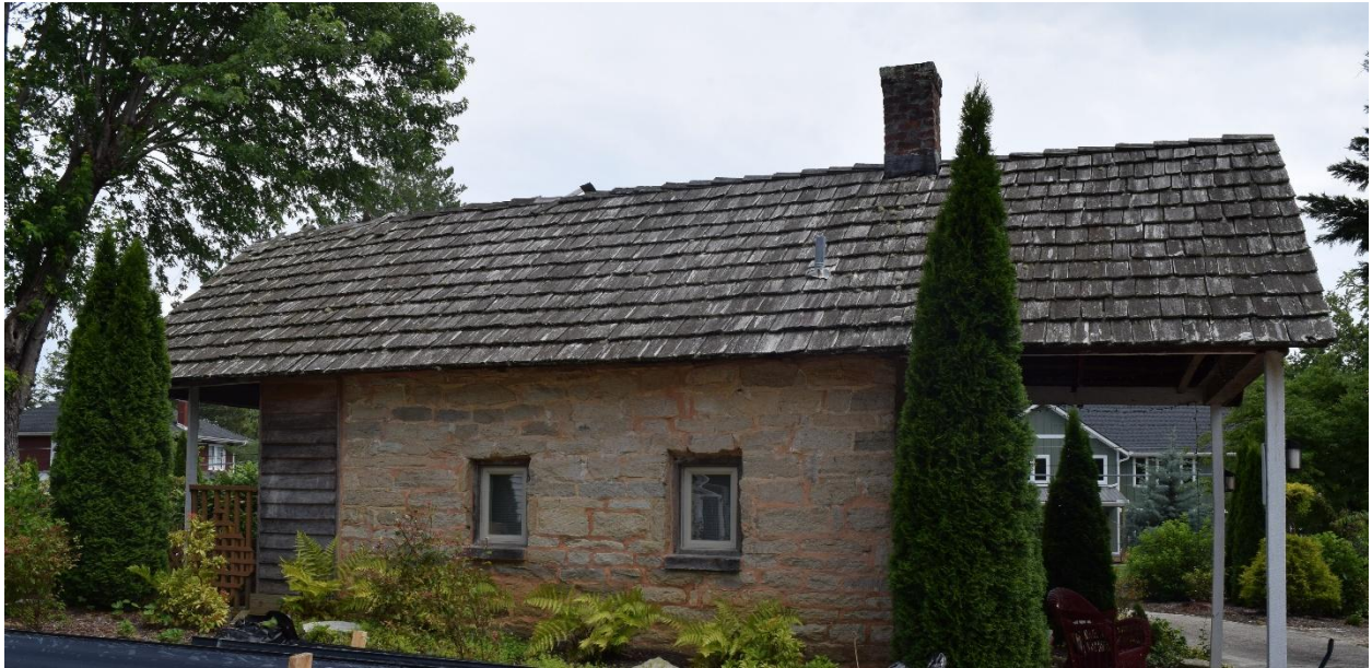
14. Carriage repair stone outbuilding, view south
