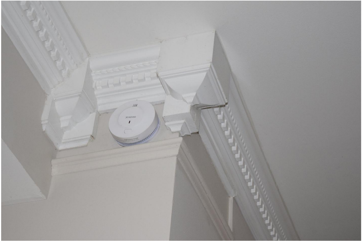
33. First floor crown molding
