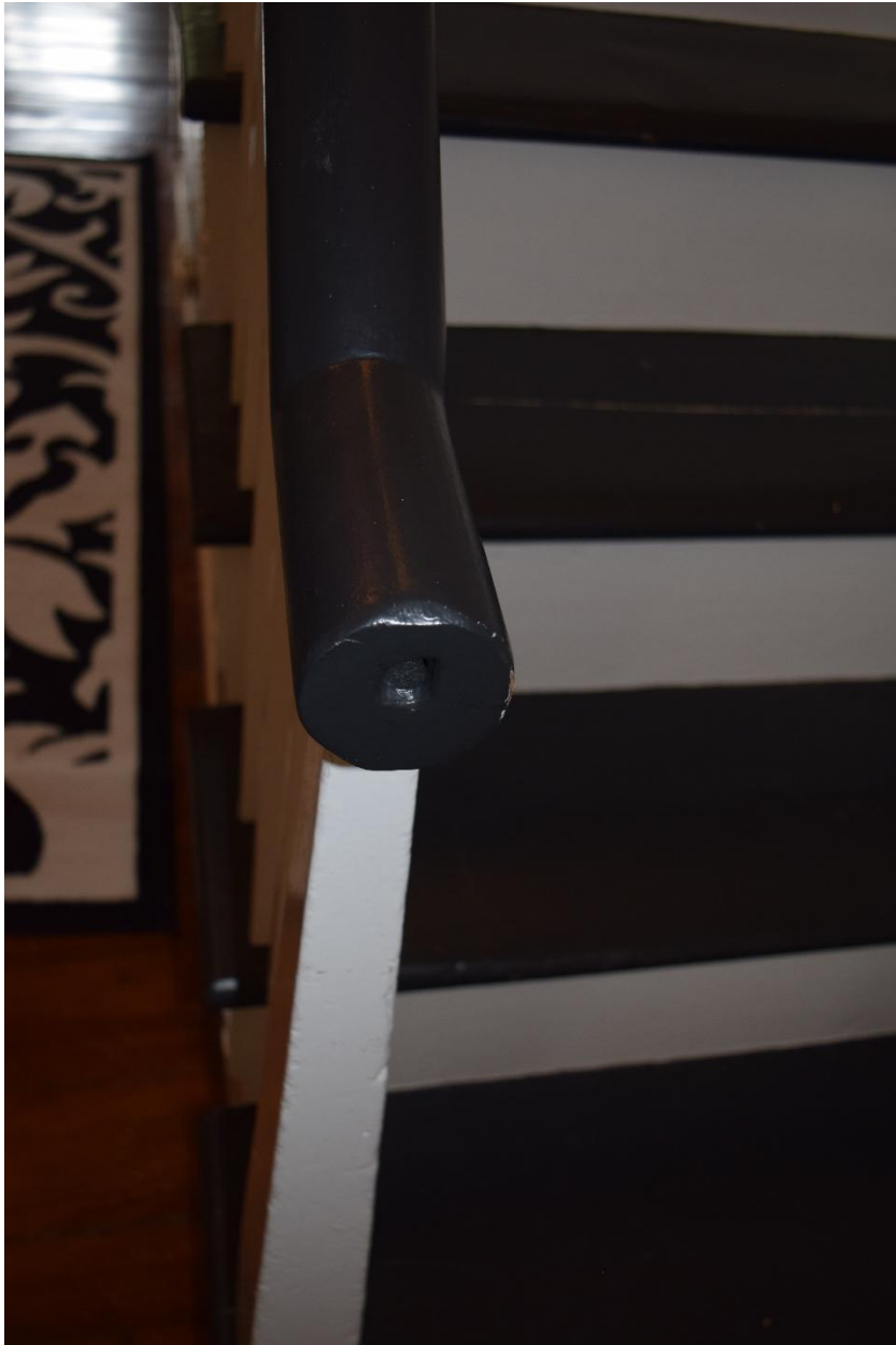
41. Banister detail, first floor staircase
