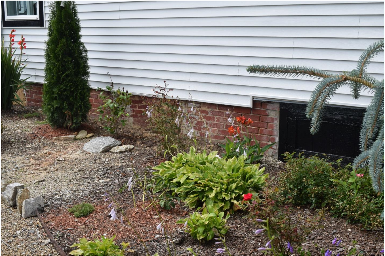
9. Brick foundation beneath kitchen wing, view northwest
