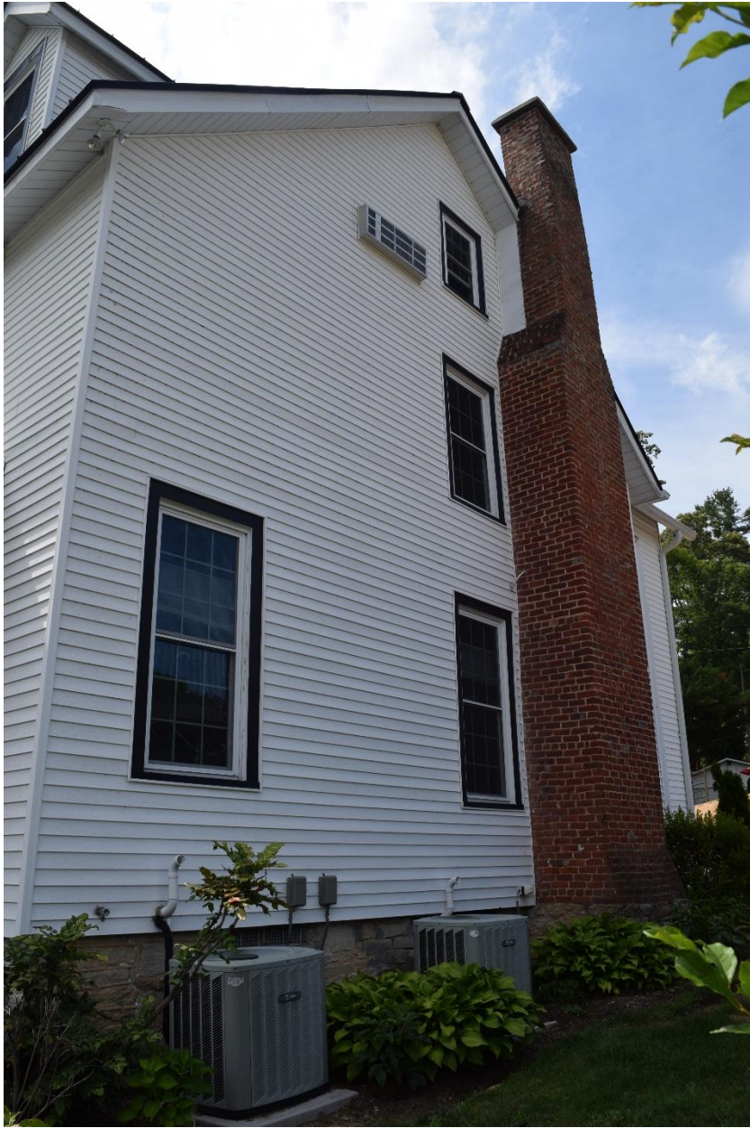
6. East elevation, view northwest
