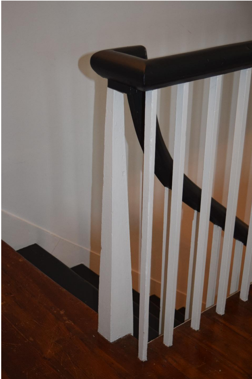
57. Second floor newel post and balustrade detail
