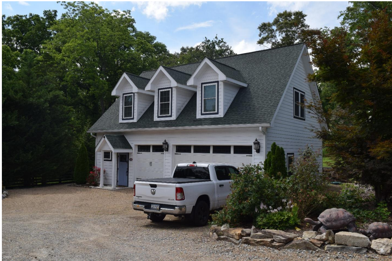
18. Non-historic garage, built 2018, view northwest
