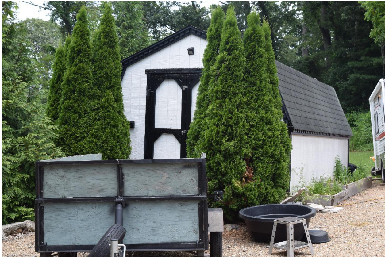
21. Non-historic storage shed, view northwest
