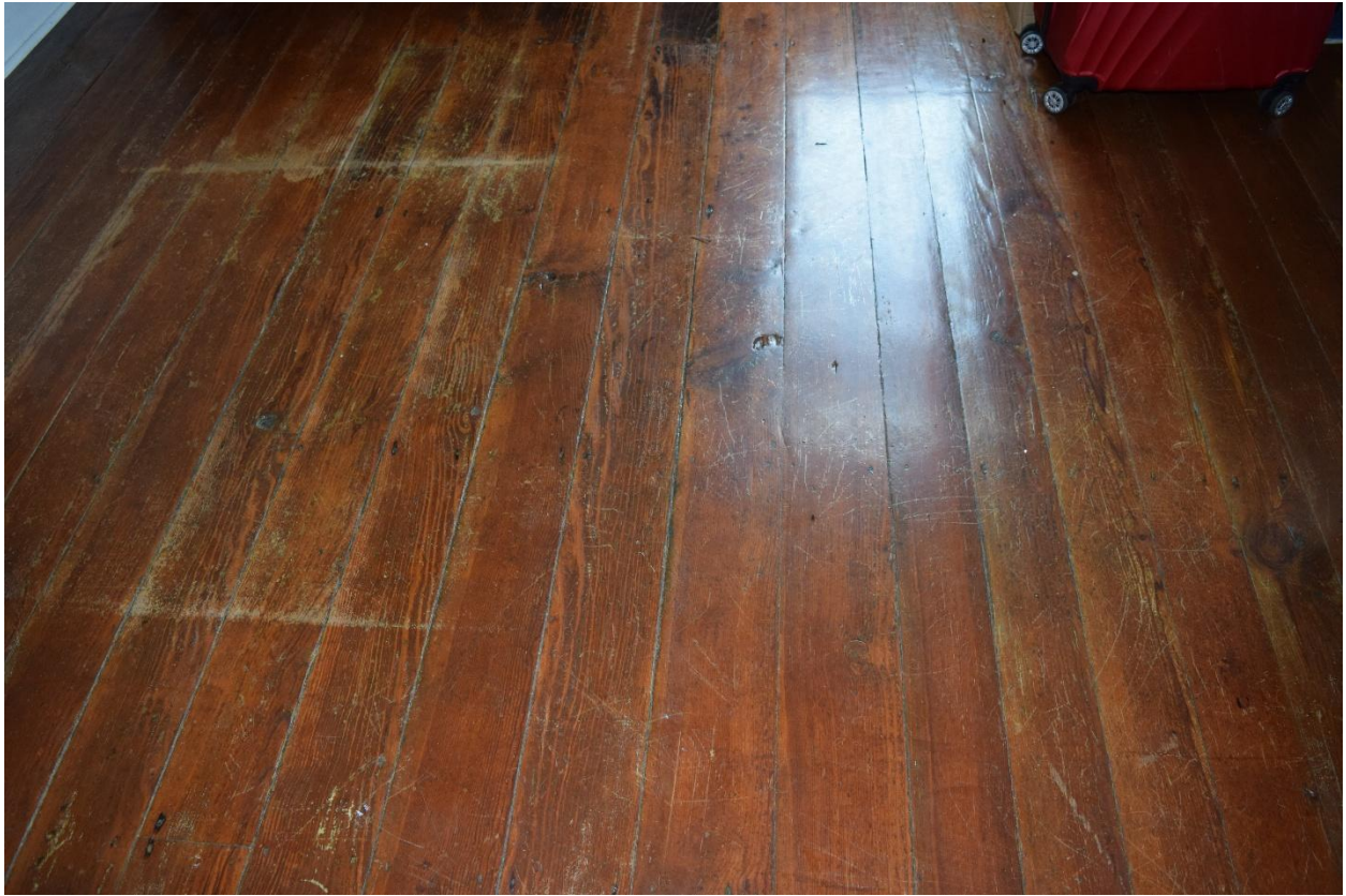
27. Wide heart pine flooring throughout the house
