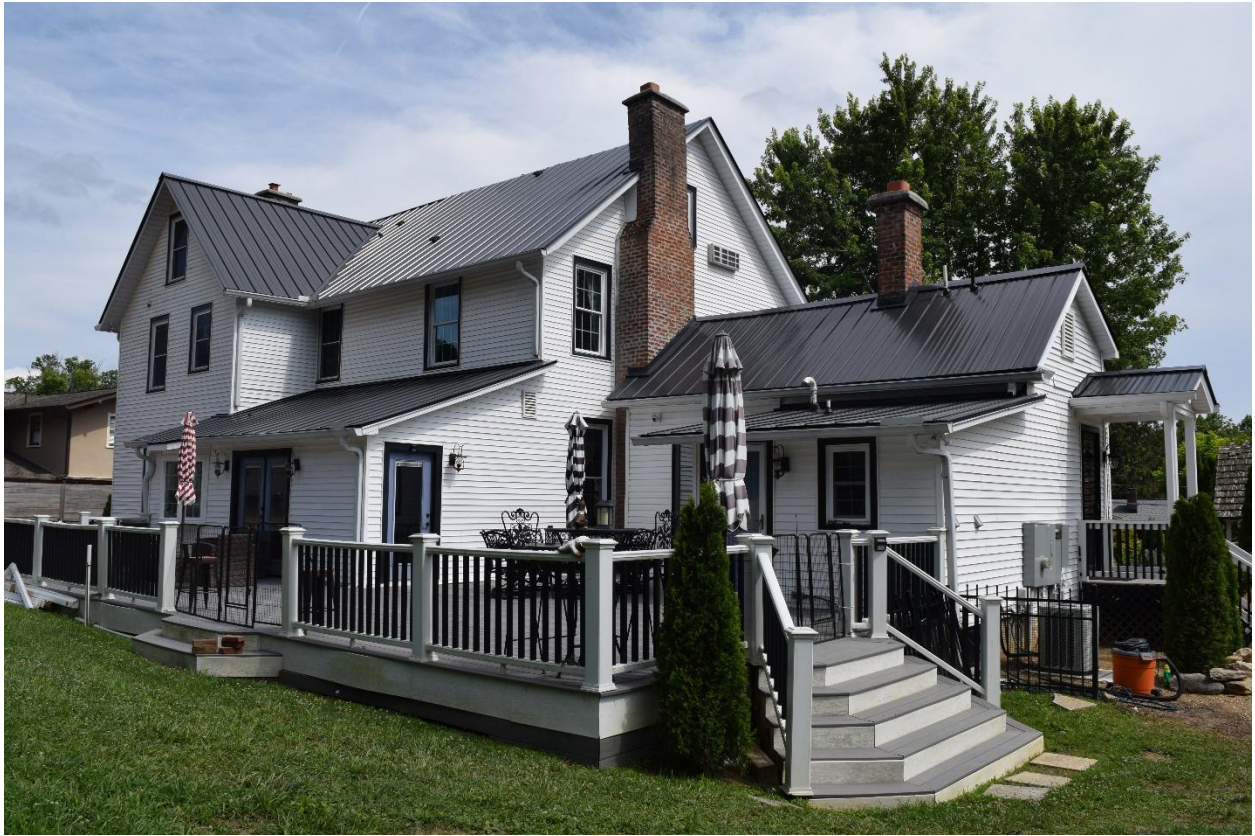
11. West elevation, view southeast
