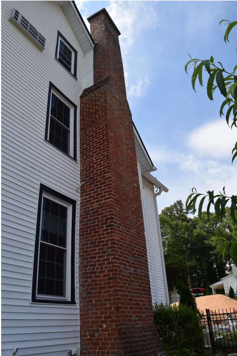
7. East elevation, single shoulder brick chimney
