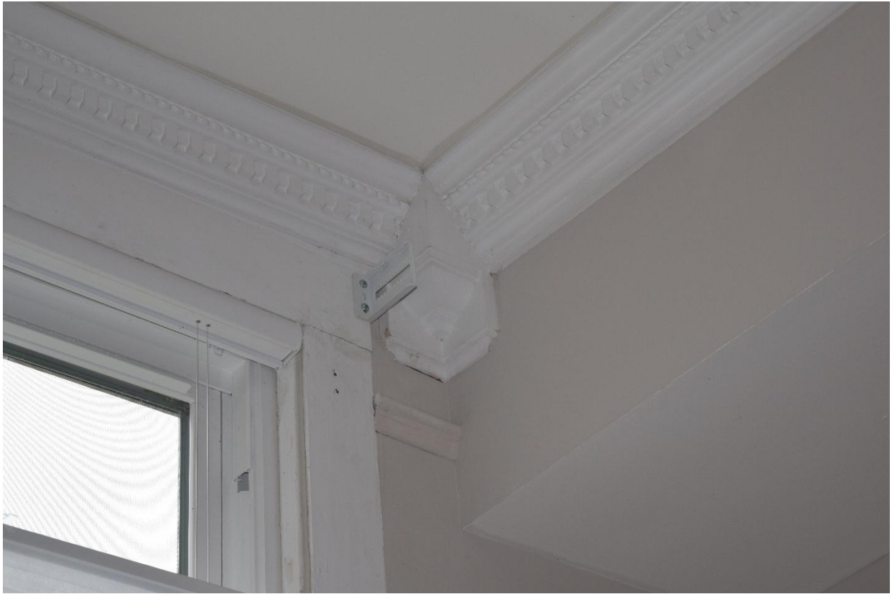
32. First floor crown molding
