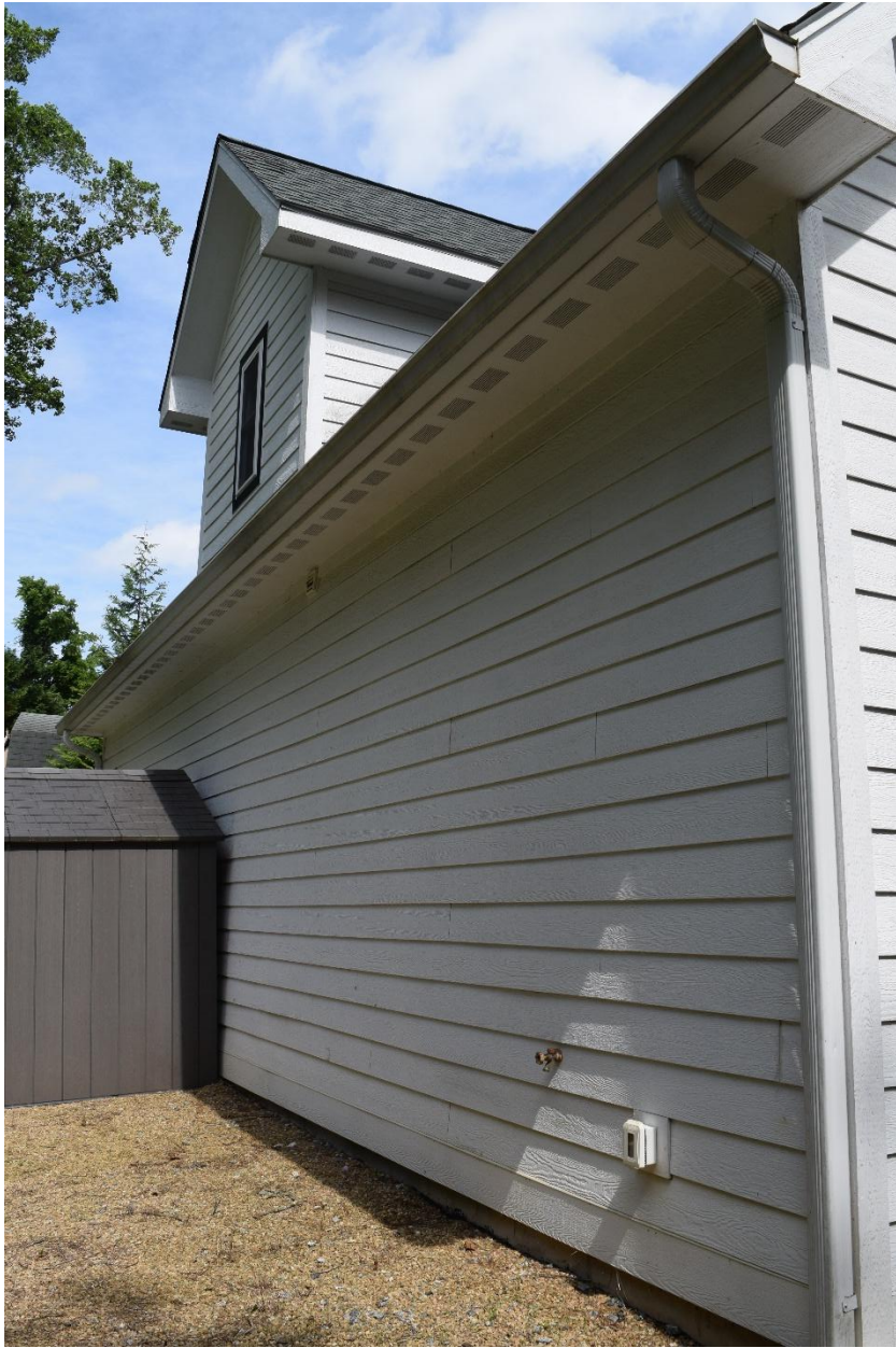
20. Non-historic garage, north elevation, view southeast
