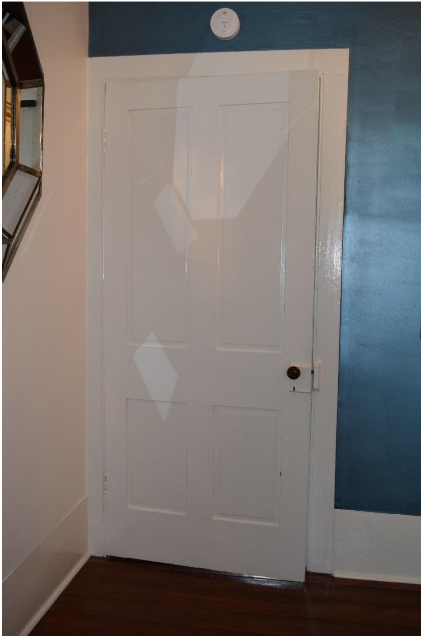
51. Typical four-panel door throughout house
