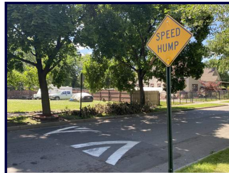
Install Speed Humps with W17-1 Signs (6 at 500' Spacing)
