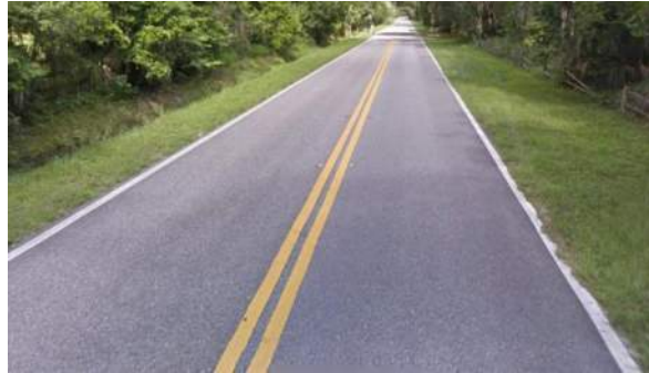
Figure 5: High-Visibility Centerline Striping
