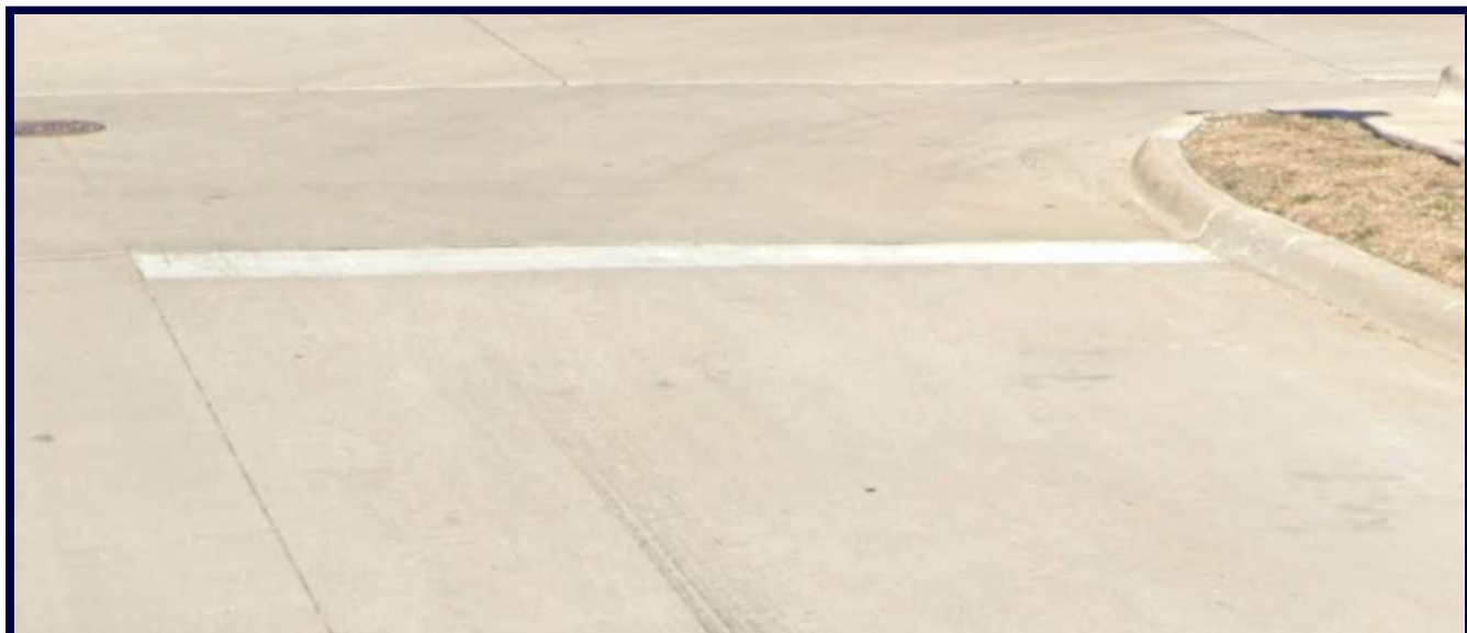
Install Stop Bar
