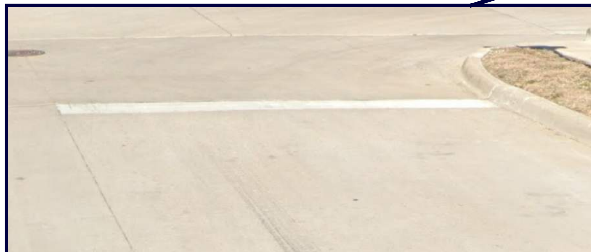
Install Stop Bar
