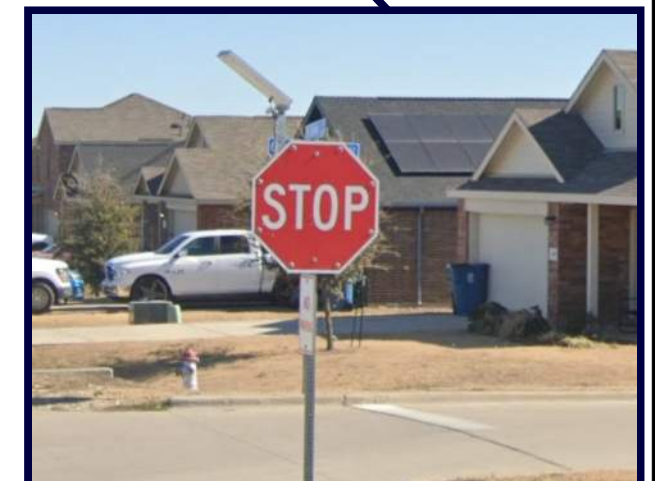
Install Stop Sign with LED Flashers
