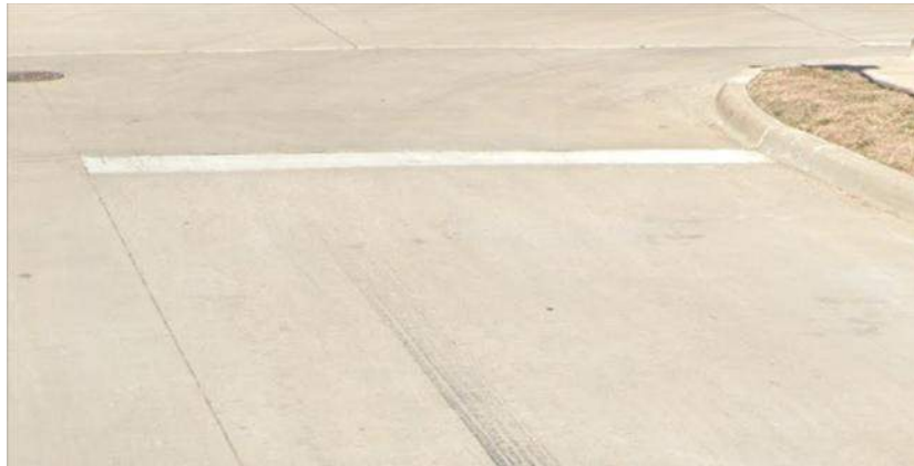
Figure 6: Stop Bar
