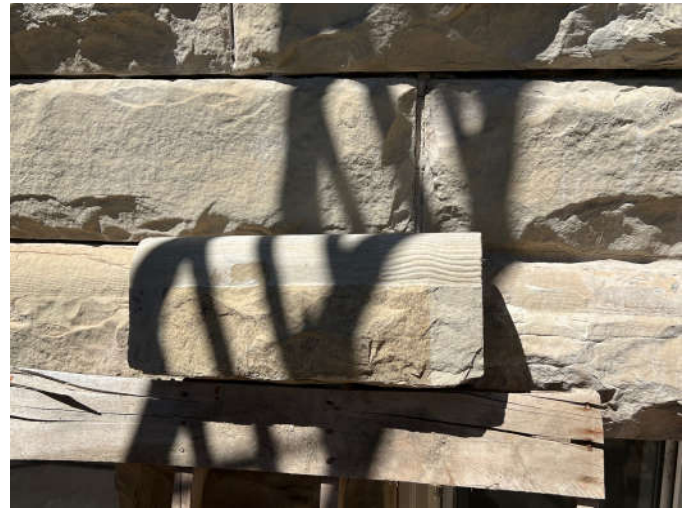
Photo #2: The stone was sandblasted at its end to match the color of the original stone more closely. A sample of the tooling at the radiused top surface of the water table stones was approved.
